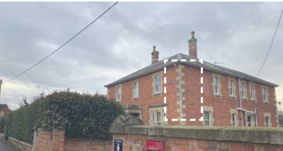
Landmark Building with Buff Stone Quoins & Hipped Roof
