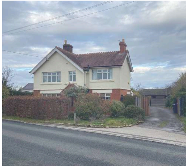
Figure 5: Split Brick and Render Elevation Detached House: Woodmarsh Road
