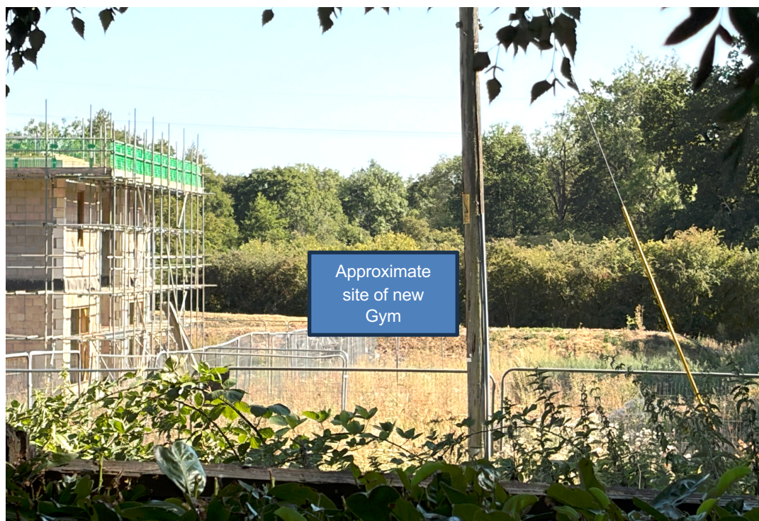
Photograph of new dwelling at Manorfield Farm from Abbotswood, 11 August 2026
