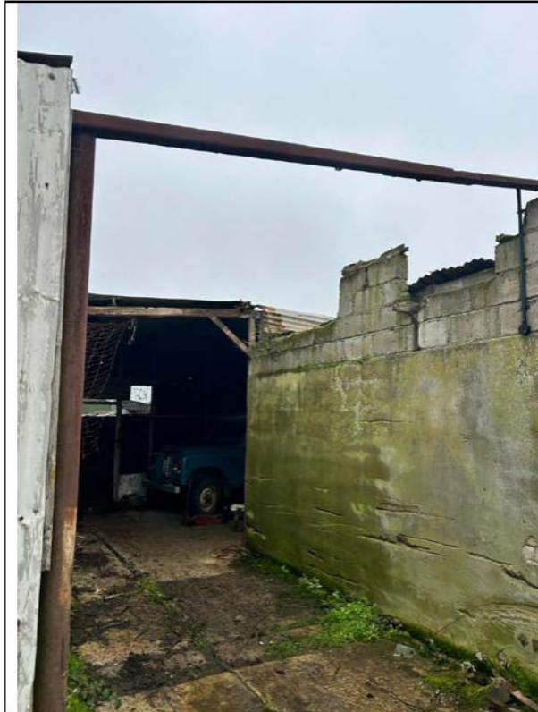
Barn 4 Front (Northern) Elevation
