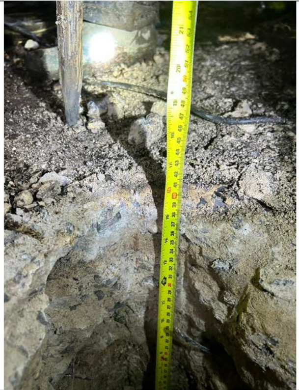
Ground Bearing Slab 400-500mm
