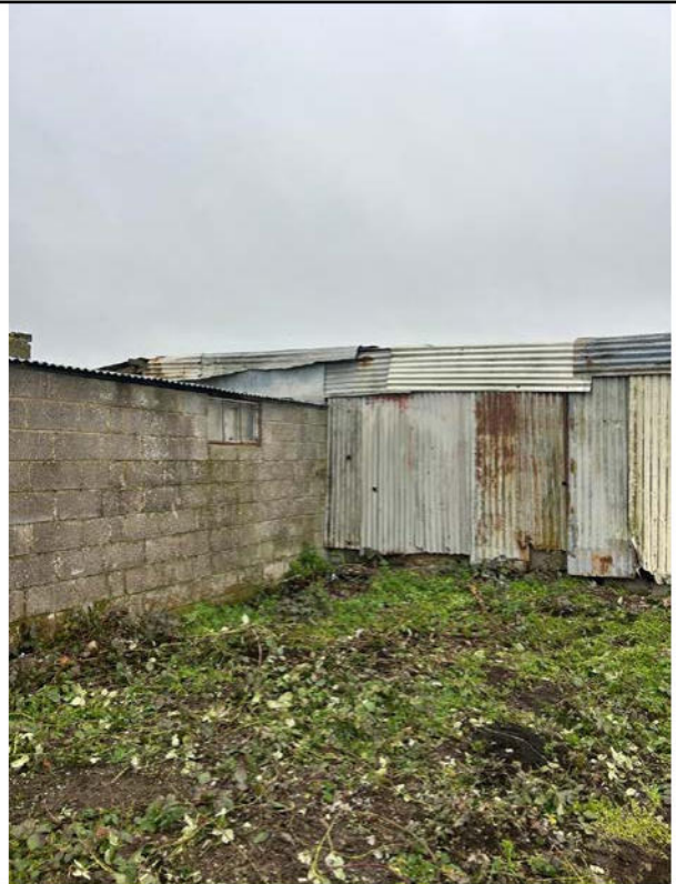
Barn 4 Rear (Southern) Elevation
