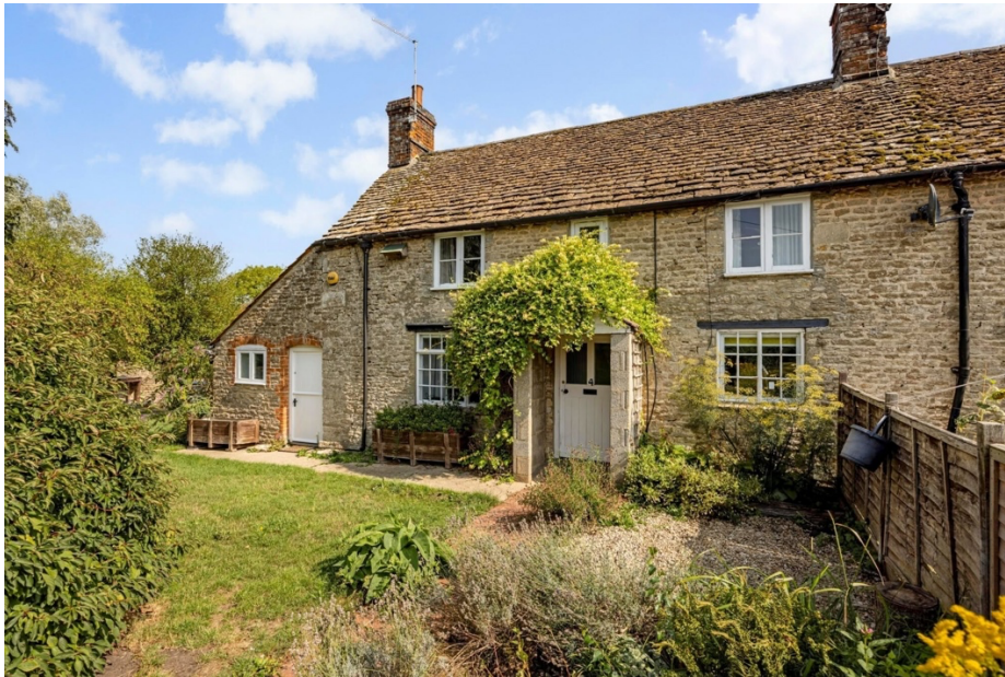
Image: Existing front (south facing) elevation. Source: butlersherborn.co.uk
