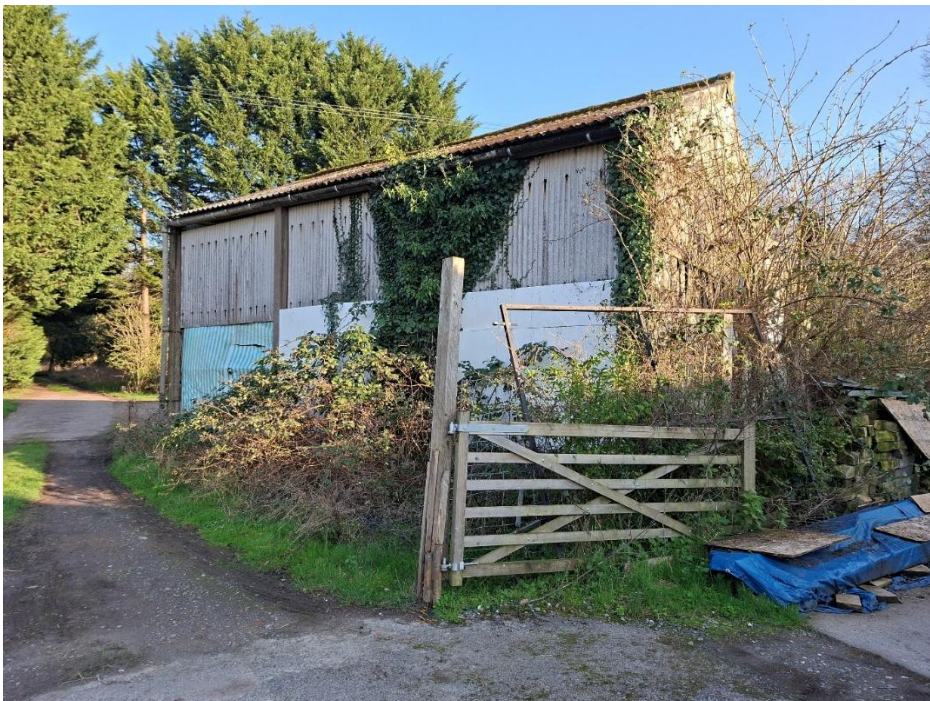
Figures 11 & 12: Views of the existing building as it previously appeared before work has taken place to continue the implementation of the Section 73 planning approval (e.g. removal of the existing roof and wall cladding)
