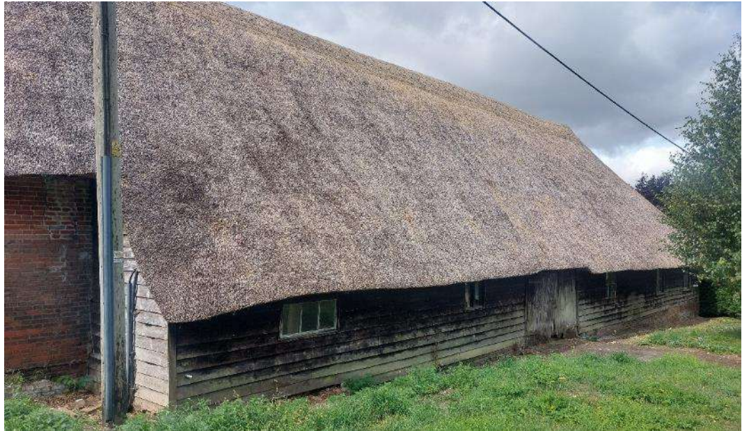
Figure 9 North elevation of the barn.
