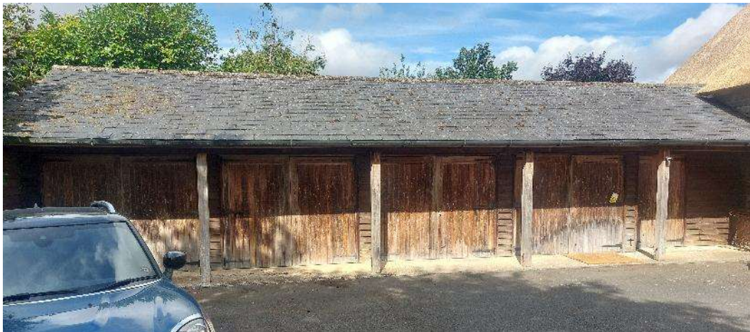
Figure 19 Garage range attached to the west end of the south elevation of the barn, east elevation.
