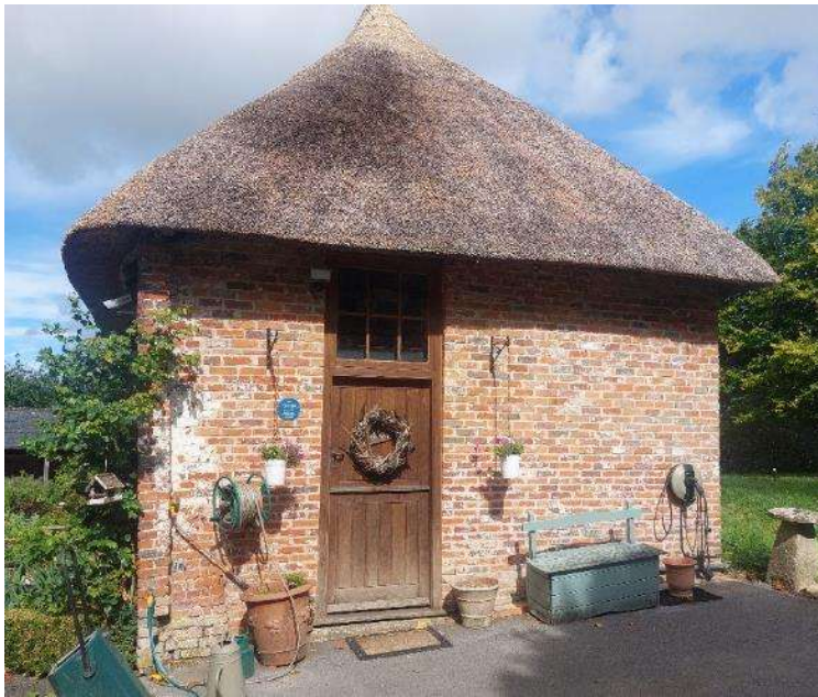
Figure 11 East elevation of the stable.
