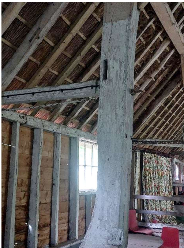
Figure 16 Void mortice for an aisle tie in the west face of the aisle post of TII for an aisle at the west end of the four-bay barn.
