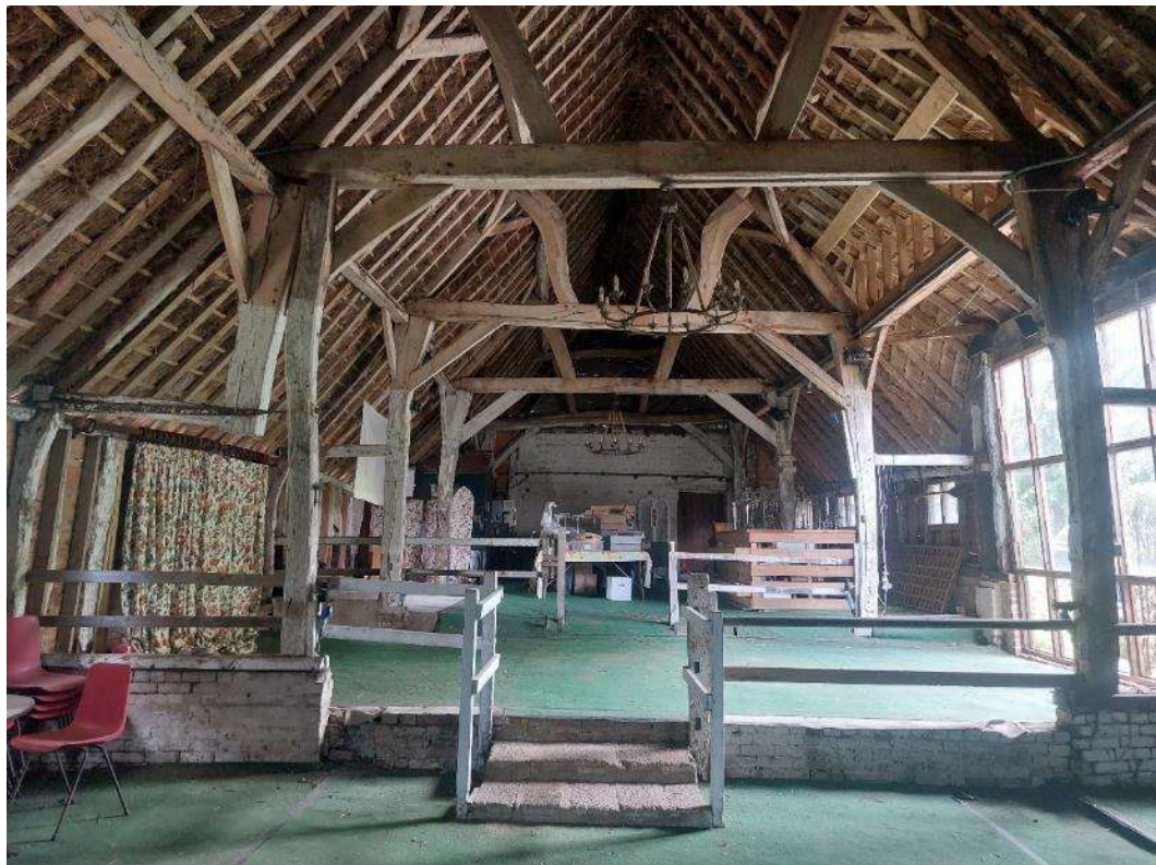
Figure 14 The interior of the barn facing east.
