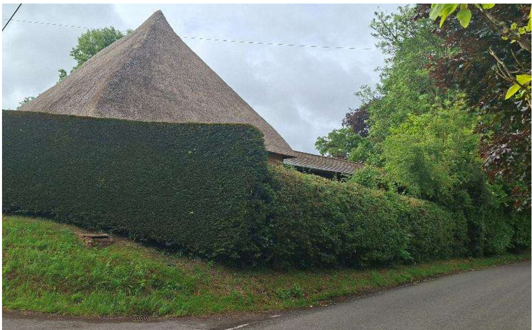
Figure 20 The barn and garage as seen from the village street.
