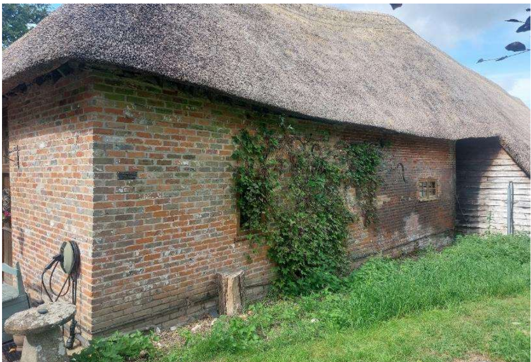
Figure 12 Rear, north elevation of the stable.
