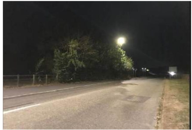
Plate 16: View east along A361 opposite the Site
