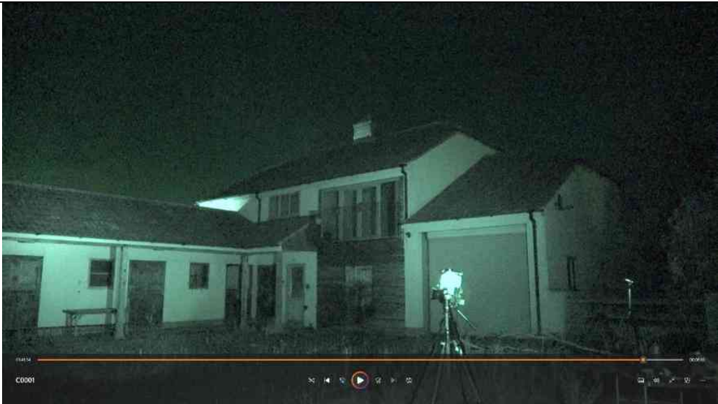
Disused Stable; south view
