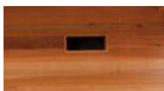
Example of bat access slot
