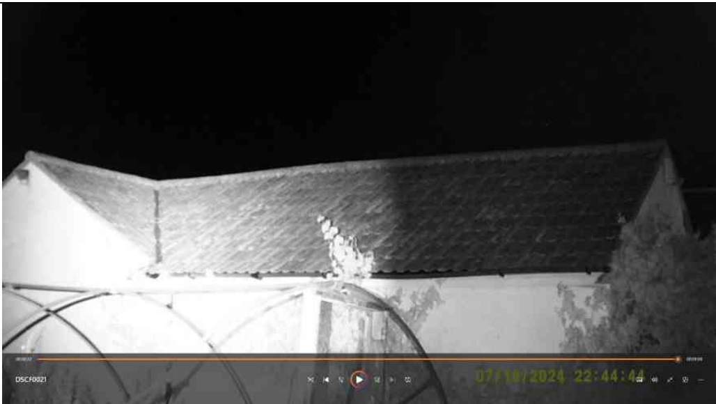
Disused Stable; south-west view
