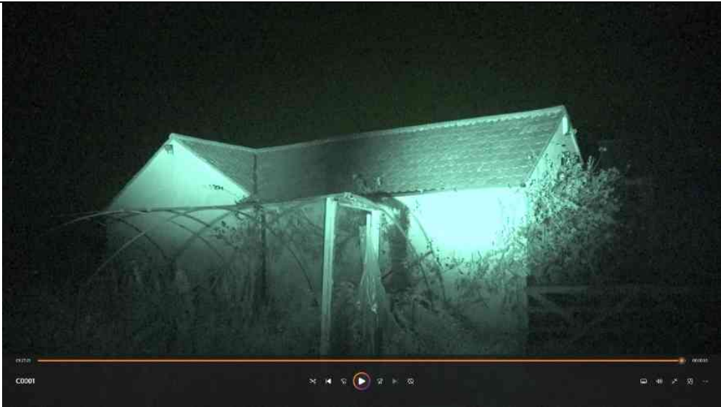
Disused Stable; south-west view
