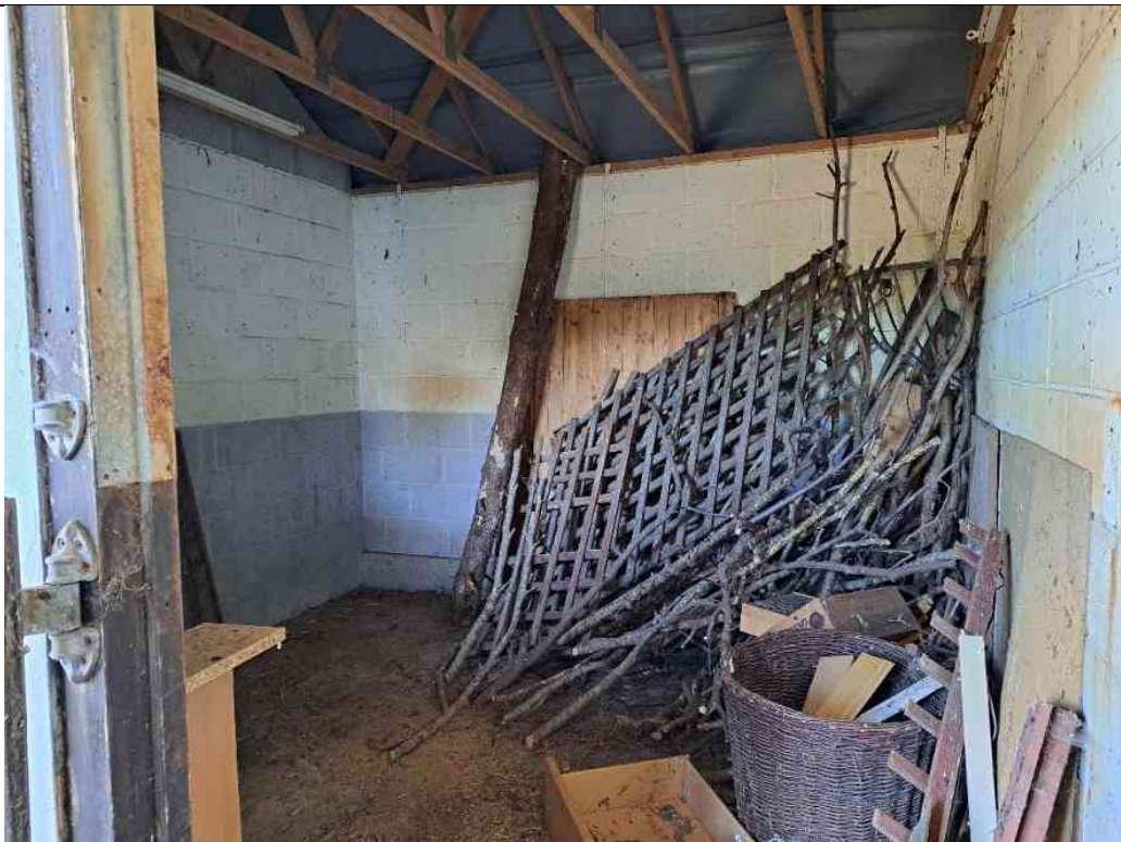
View looking into the open stable unit of the Disused Stable
