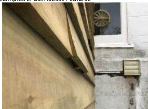
Example of cladding based crevice roost
