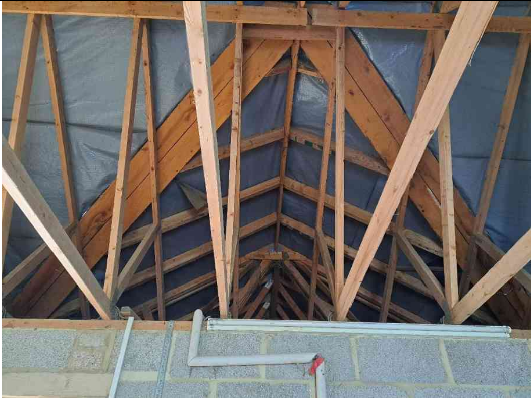
Open roof void above stable kitchen of Disused Stable
