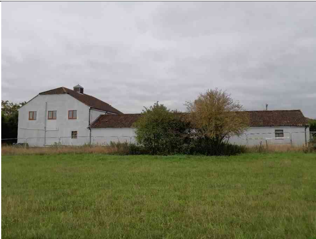
North view of Disused Stable
