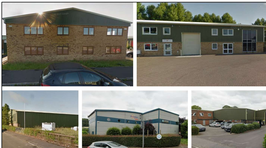
Figure 2: Collage showing form and materiality common across Downton Business Park Principal Employment Area, courtesy of Google Street View
