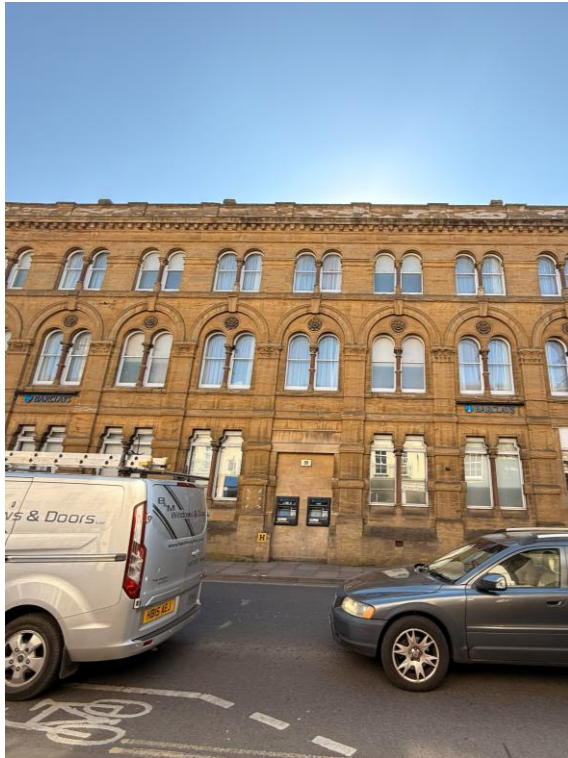
Photograph 1 – Location of external ATMs
