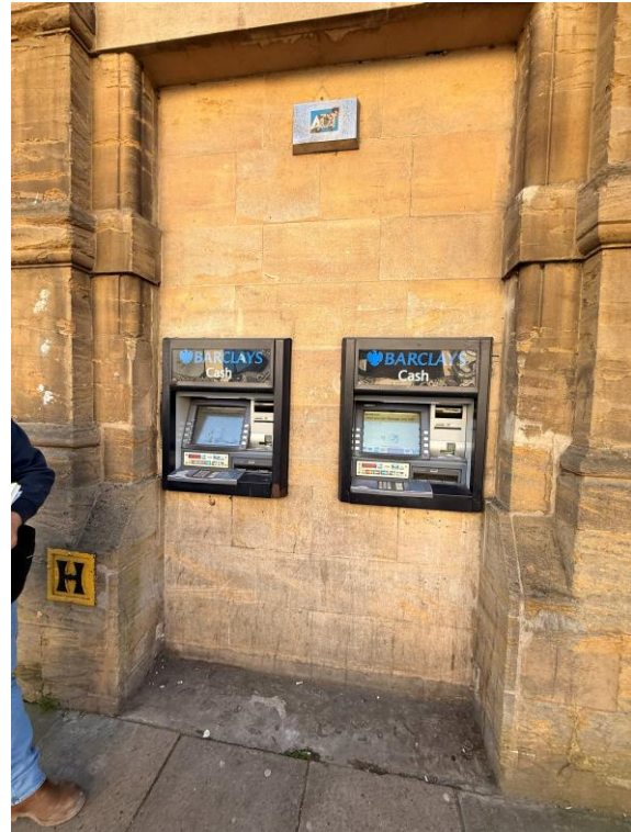
Photograph 2 – Existing external ATMs
