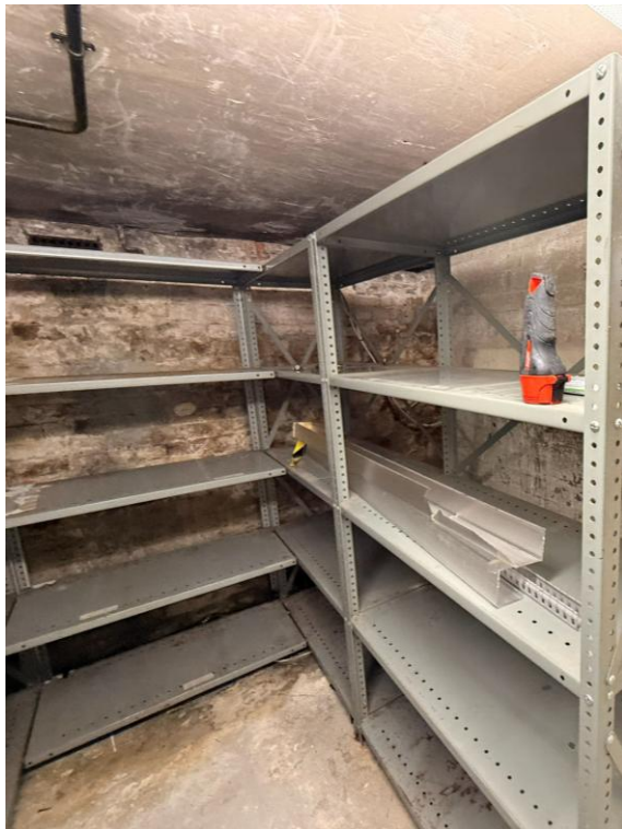
Photograph 7 - Basement, internal view of north elevation, view 2
