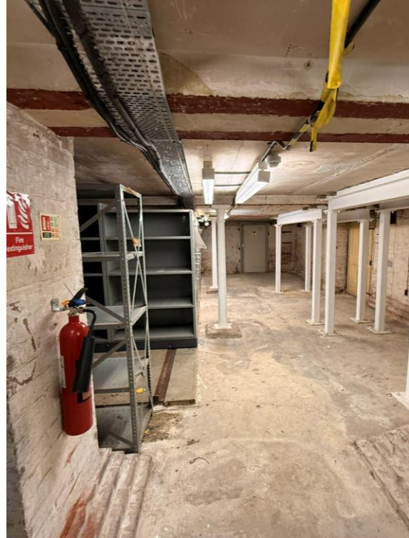
Photograph 6 – Basement, easterly view
