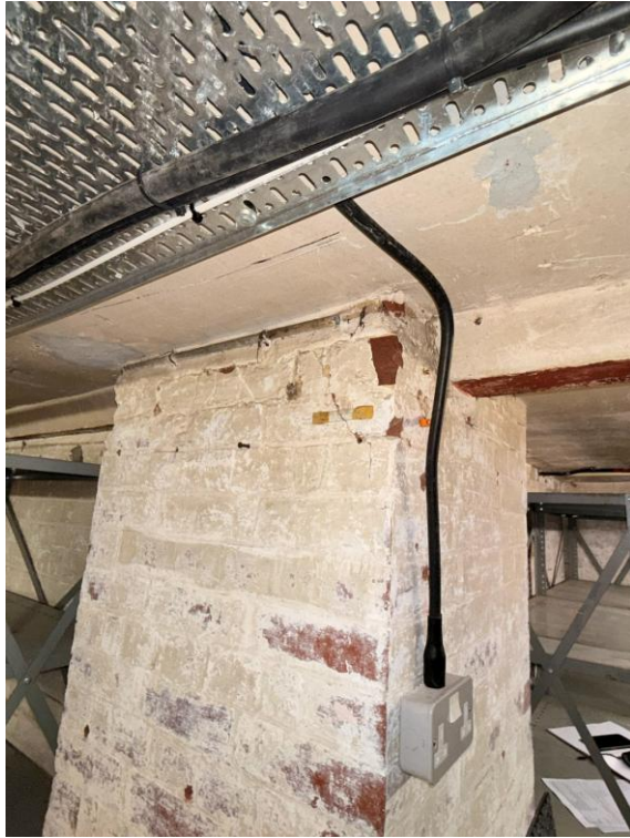
Photograph 5 – Basement, masonry pier supporting structural beams
