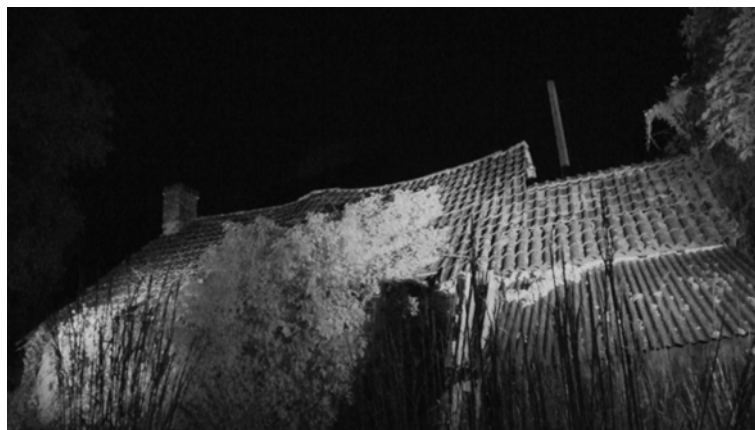
Figure 1: Still from Infra-Red camera on eastern elevation.
