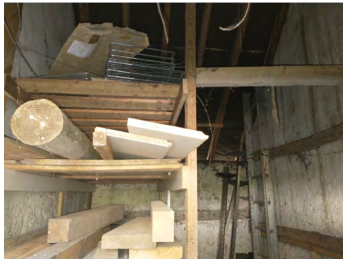
Figures 19: Interior of shed section.
