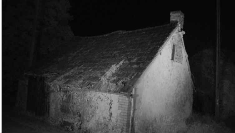
Figure 2: Still from Infra-Red camera of southwest aspect.
