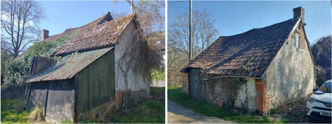
Figures 14 and 15: Old Forge building from northeast aspect and southwest aspect, respectively.
