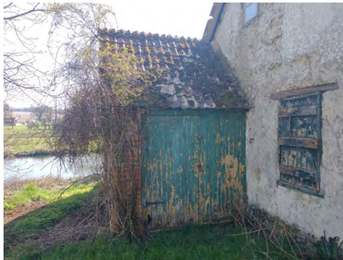
Figure 16: Shed extension on northern elevation.
