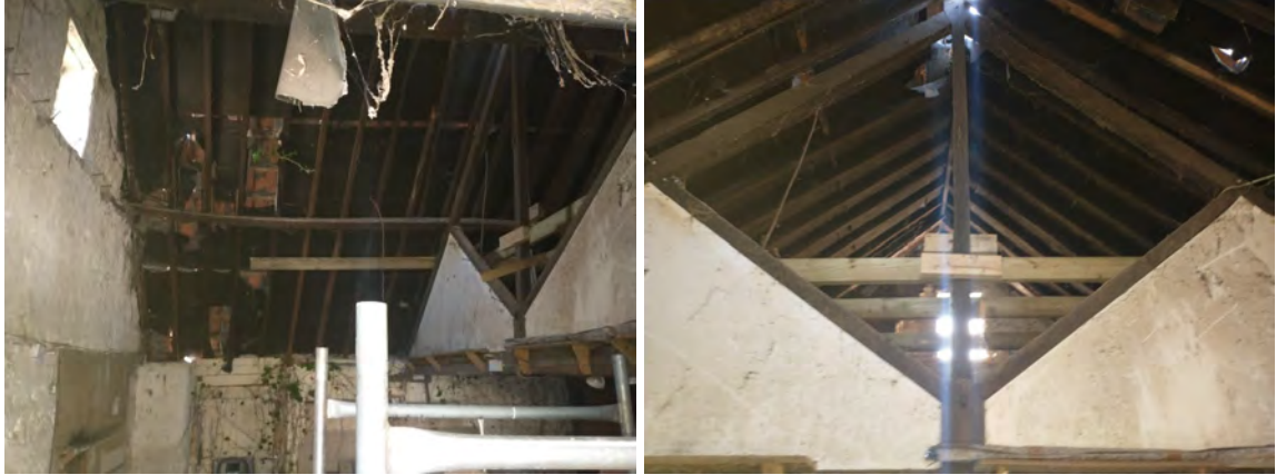
Figures 17 and 18: Interior of building.
