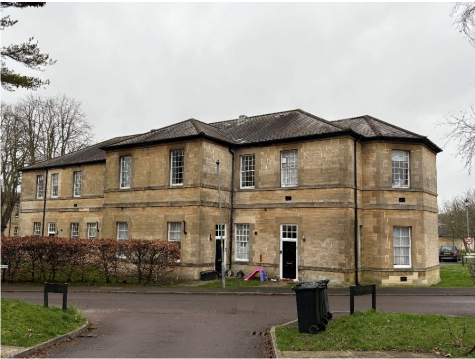
Photograph of Northwest elevation (Savills UK, 2026)
