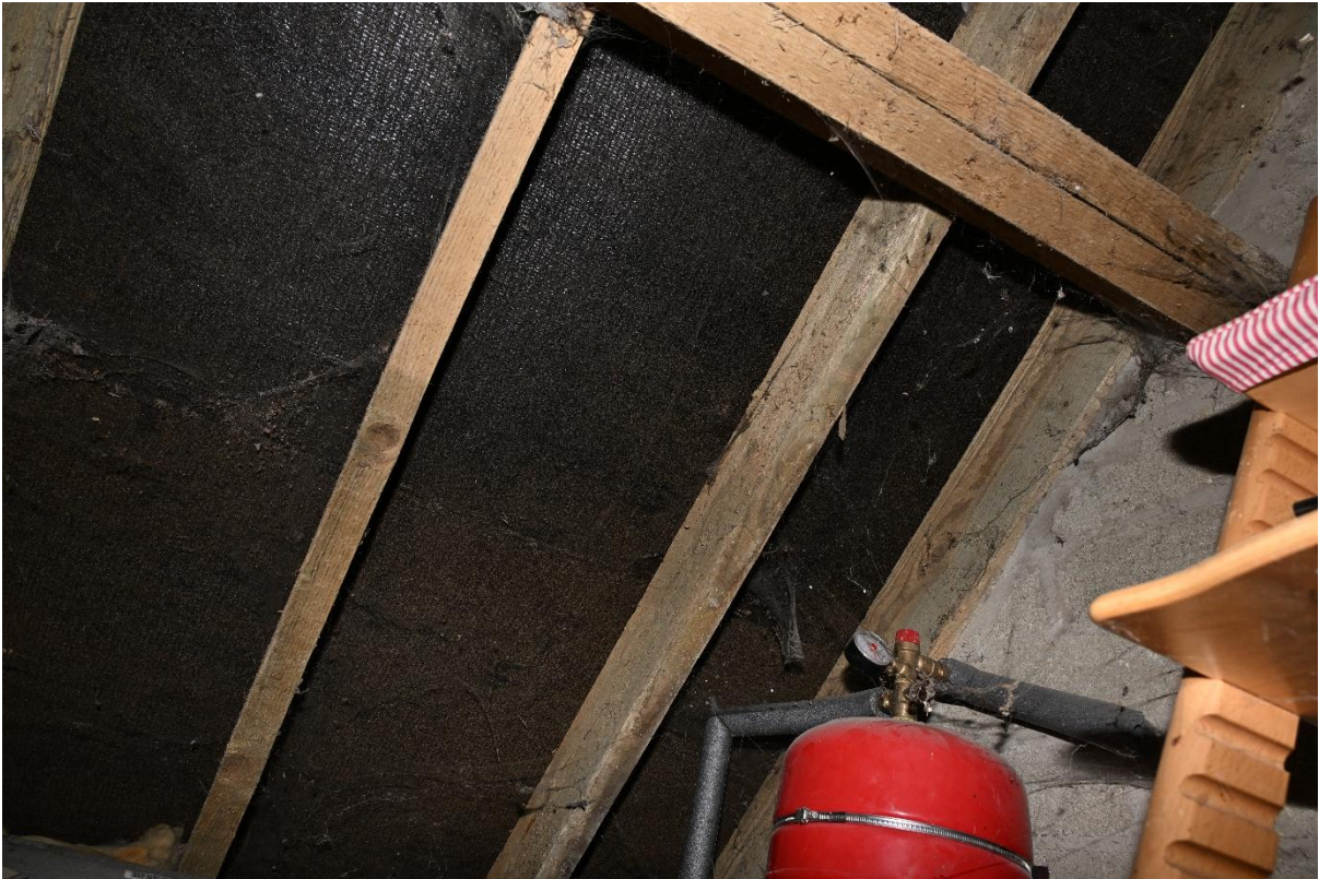
Image 5 Roof structure and underfelt
