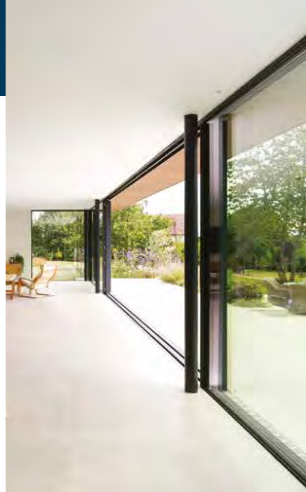
SL700 track with matching flush floors inside and out
