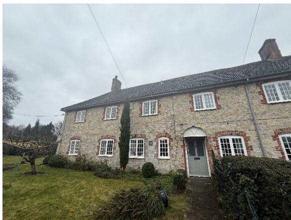
Front of B1 – NW Elevation
