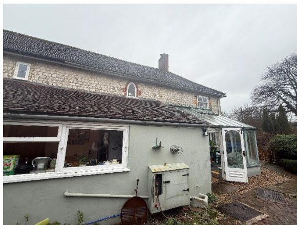
South-East Elevation of B1 facing East
