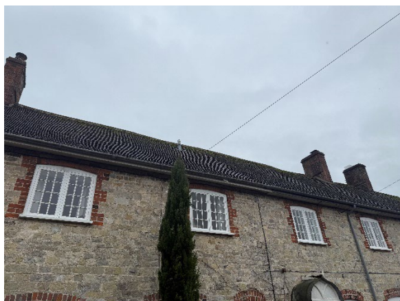
Roof line of the front of B1 (West Elevation)
