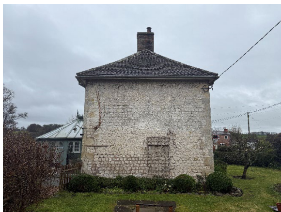
Northern elevation of B1, facing South
