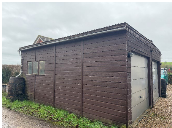
North elevation of B2 (Garage Building)
