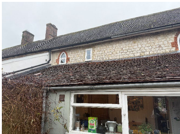
South-East Elevation of B1 facing West
