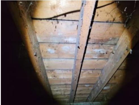
Photo 7: Wooden boarding beneath tiles.
