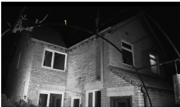
Image 1: End of survey Image. Survey 1 20/05/26
