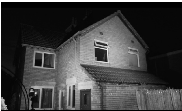
Image 5: End of survey Image. Survey 3 07/07/26
