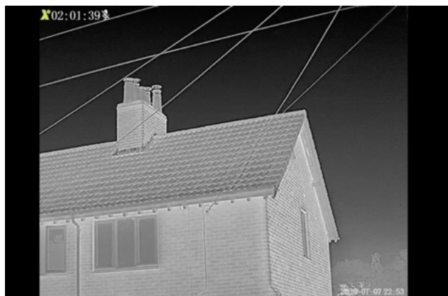
Image 6: End of survey Image. Survey 3 07/07/26
