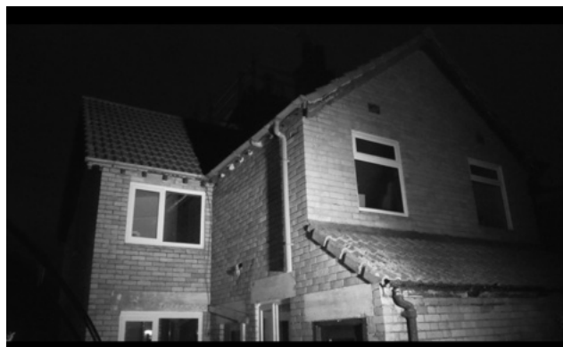
Image 4: End of survey Image. Survey 2 15/06/26
