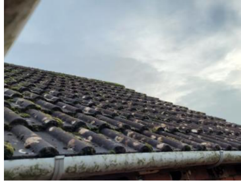
Photo 2: Well fitted concrete interlocking tiles.
