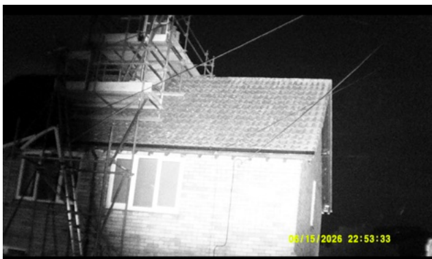
Image 3: End of survey Image. Survey 2 15/06/26
