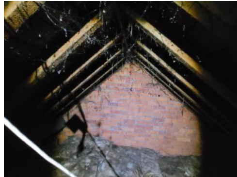
Photo 6: An internal view of the loft void.
