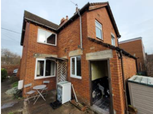
Photo 1: View of the building from the south-west.
