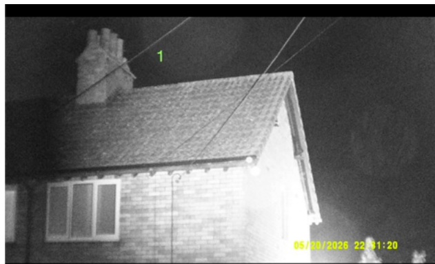
Image 2: End of survey Image. Survey 1 20/05/26
