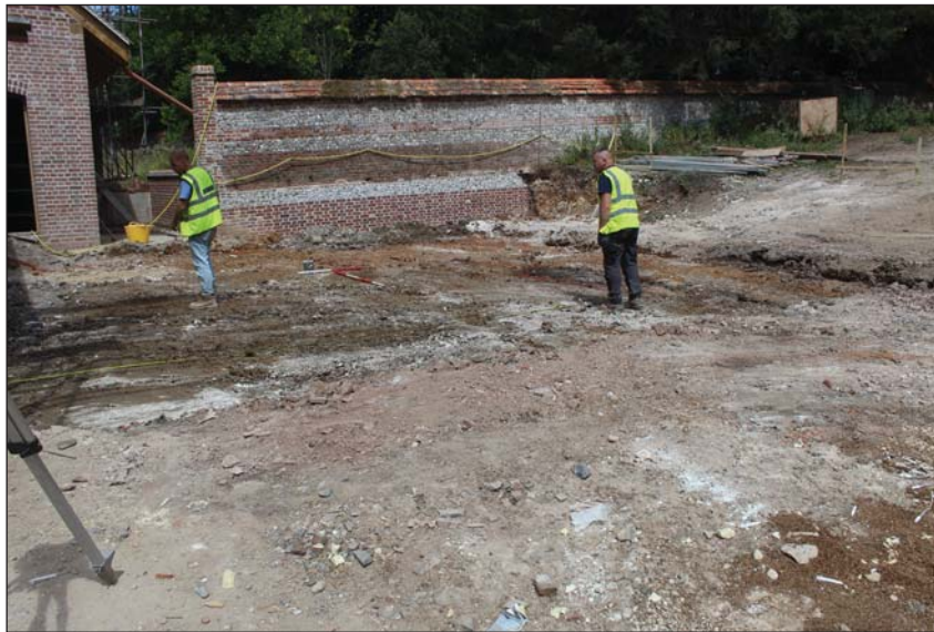
Plate 1. Ground reduction area looking north west, Scales: 2m and 1m
