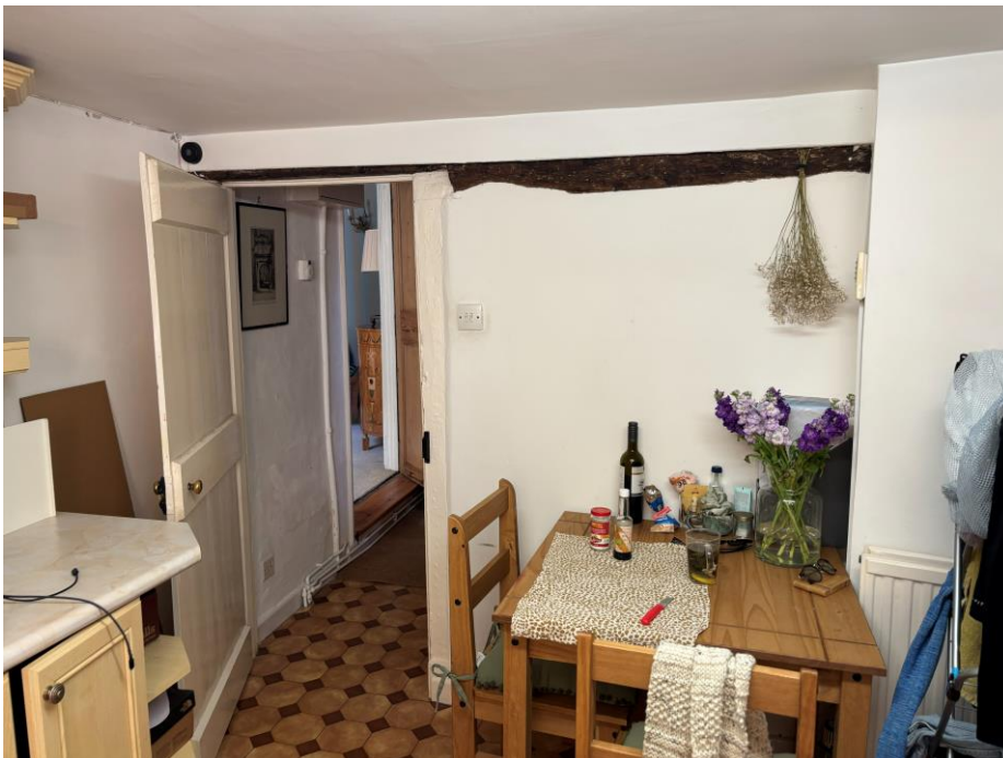
Fig.17 Former coalhouse and 'cellar' – exposed element of timber frame in the partition
