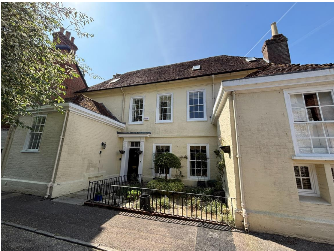
Fig.2 Front (east) elevation of 25 The Close
