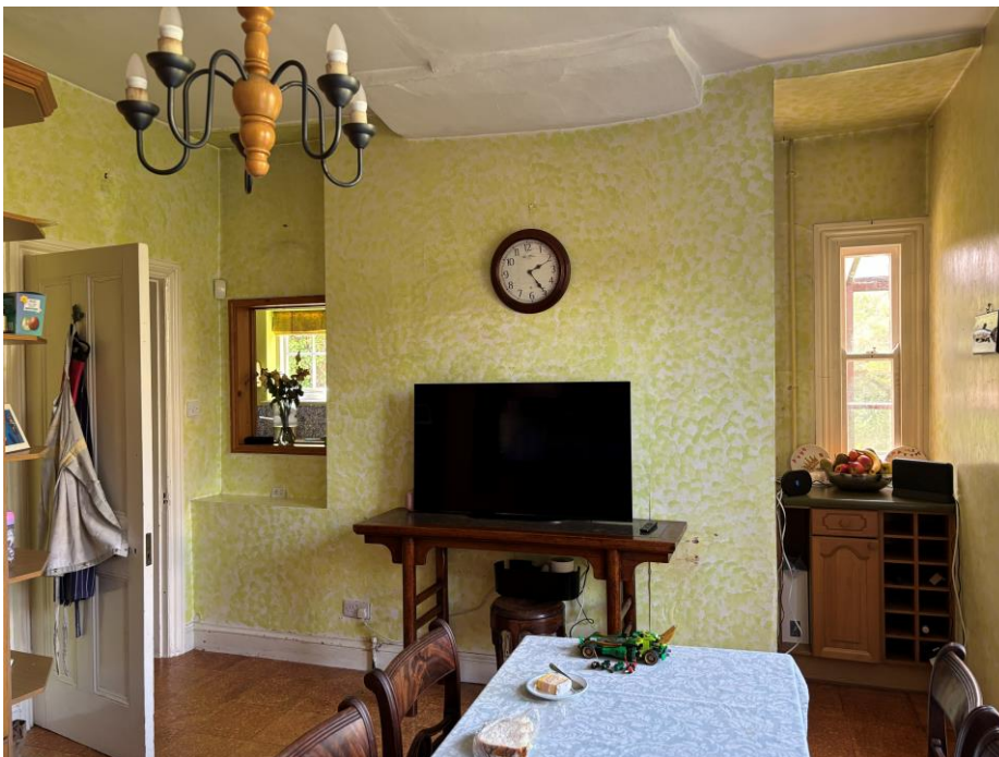
Fig.13 West wall of the kitchen
