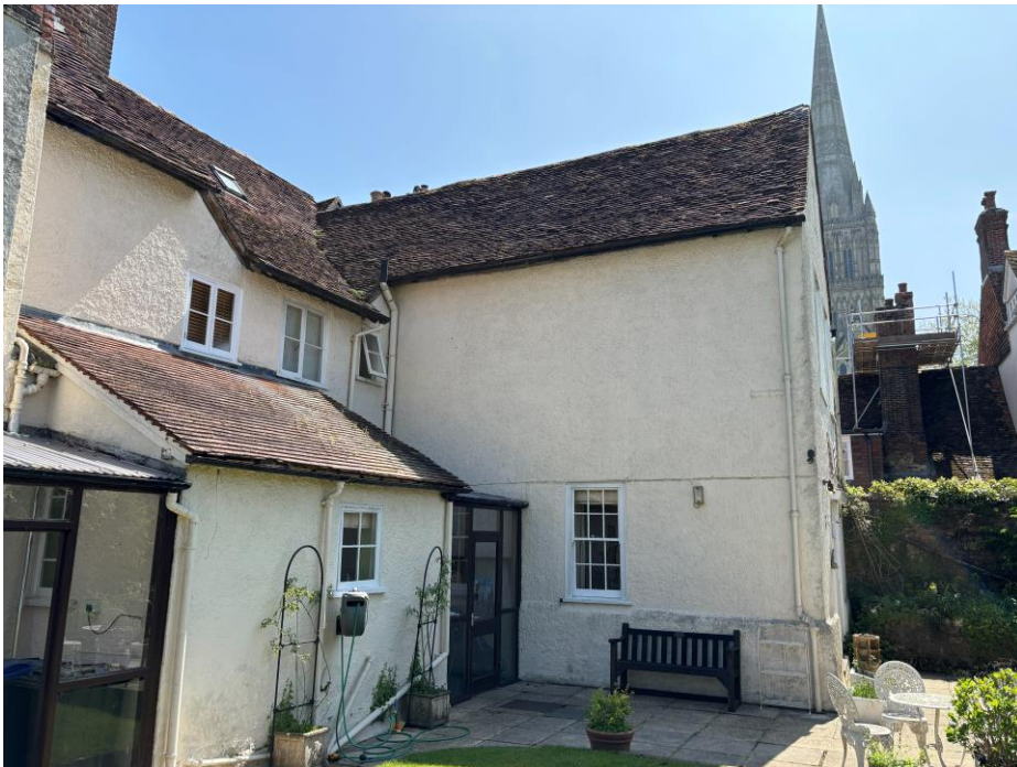
Fig.4 Back of the house with 2-storey projection and single-storey additions
