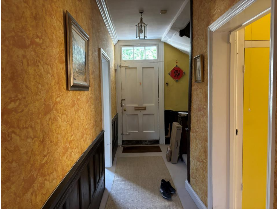
Fig.8 Entrance hall – wainscot to north wall
