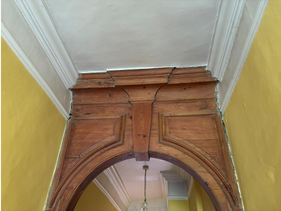
Fig.18 Panelled archway on the approach to the rear bedroom on the first floor
