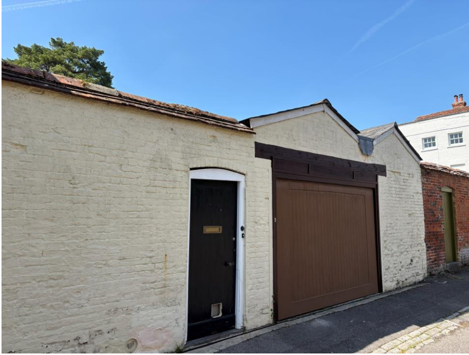
Fig.3 Wall on Rosemary Lane enclosing the rear garden; attached garage and shed
