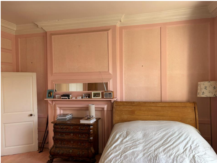
Fig.19 Rear bedroom having a deep cornice and C18 panelling and bolection-moulded fireplace, and two-panel door to the en-suite bathroom
