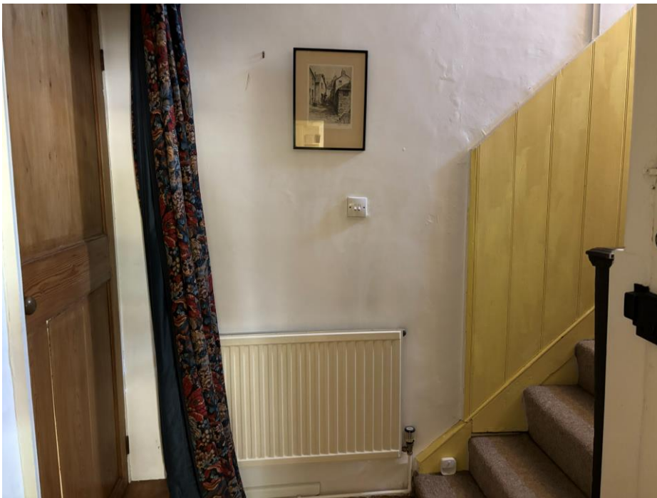
Fig.15 Blocked doorway from the northern stair hall
