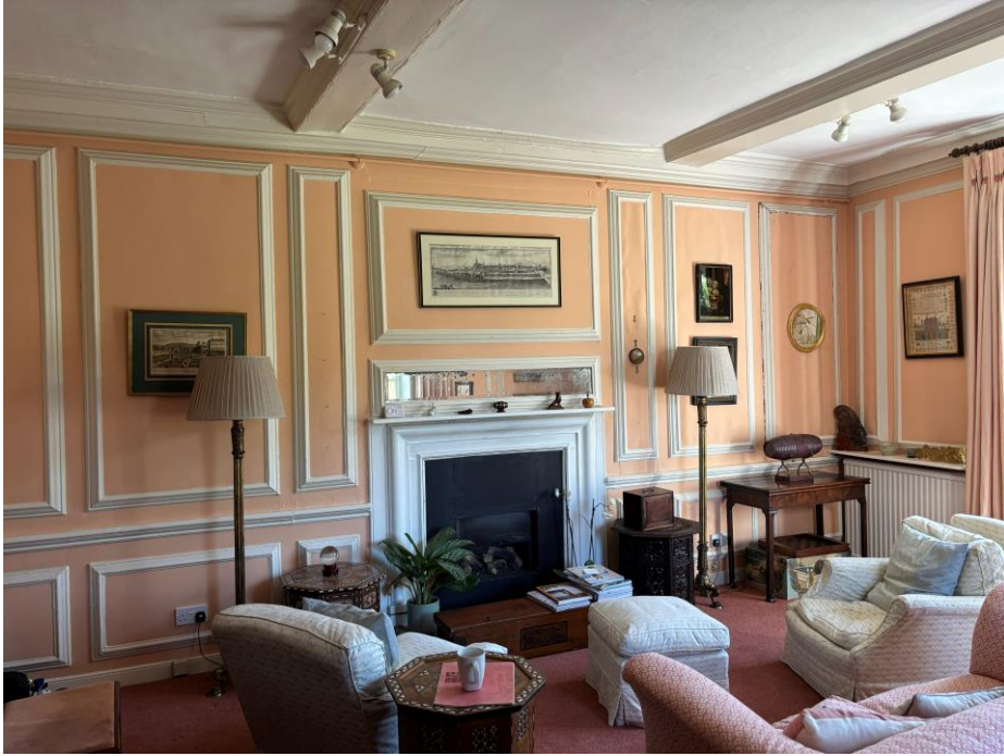
Fig.10 Dining Room with bolection-moulded panelling and fire surround
