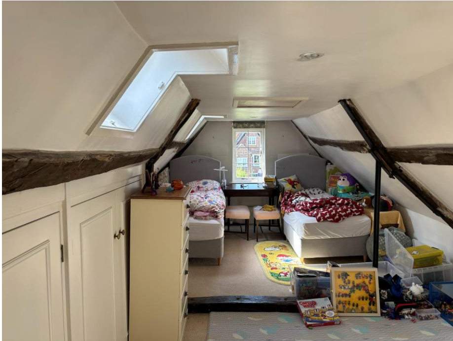
Fig.22 Attic room within south-western corner of the house with exposed elements of the C18 roof and a plasterboard ceiling
