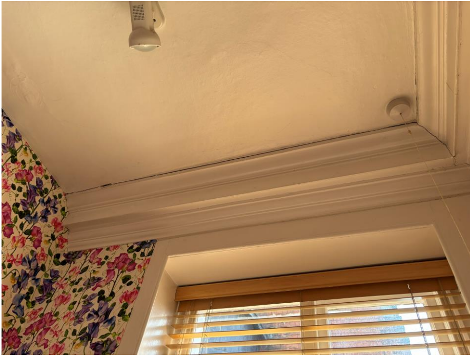
Fig.20 Partition cutting across the cornice in the en-suite bathroom
