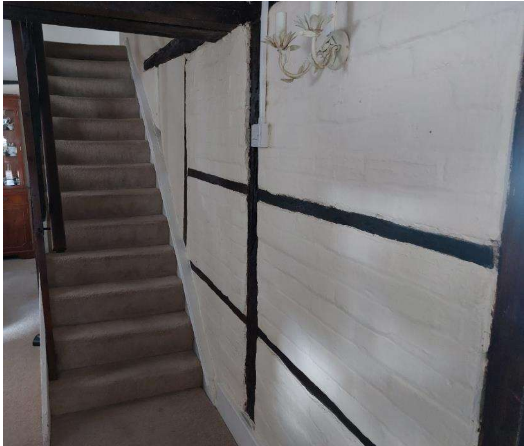
Figure 18 The modern stair within the rear wing with the lacing timbers in the rear wall of the main block of the house. One set of panels adjacent to the stair is rendered and may represent the presence of a blocked door.
