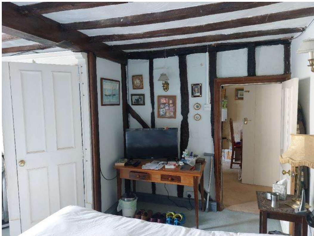
Figure 13 The south wall of the northern principal room at ground floor level.
