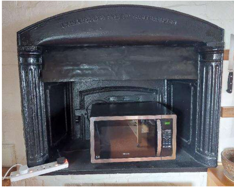
Figure 17 The cast iron front to the bread oven, made by Lancaster & Son Ltd., Southampton.
