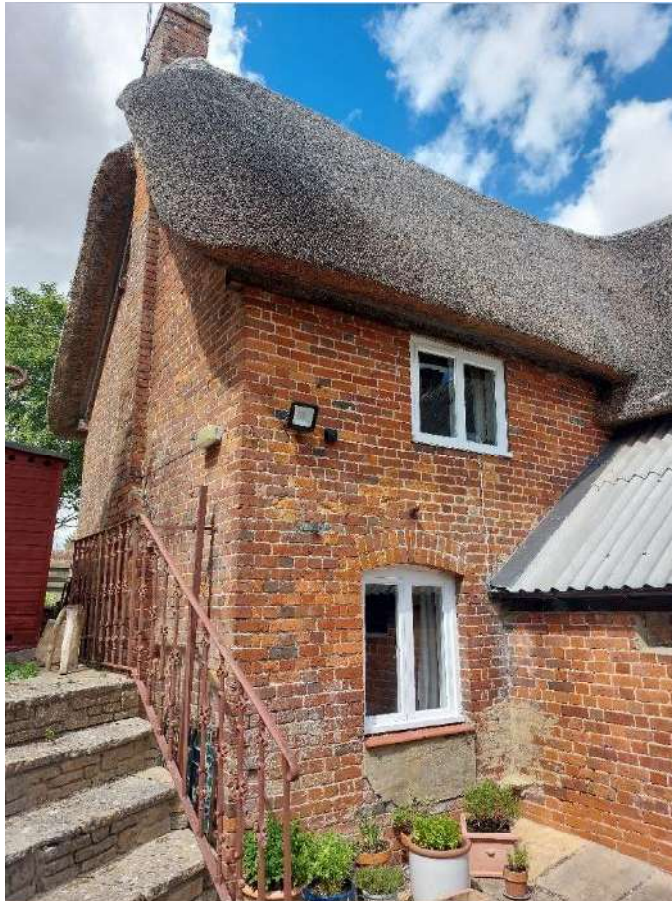
Figure 8 The southern flank wall of the rear wing.
