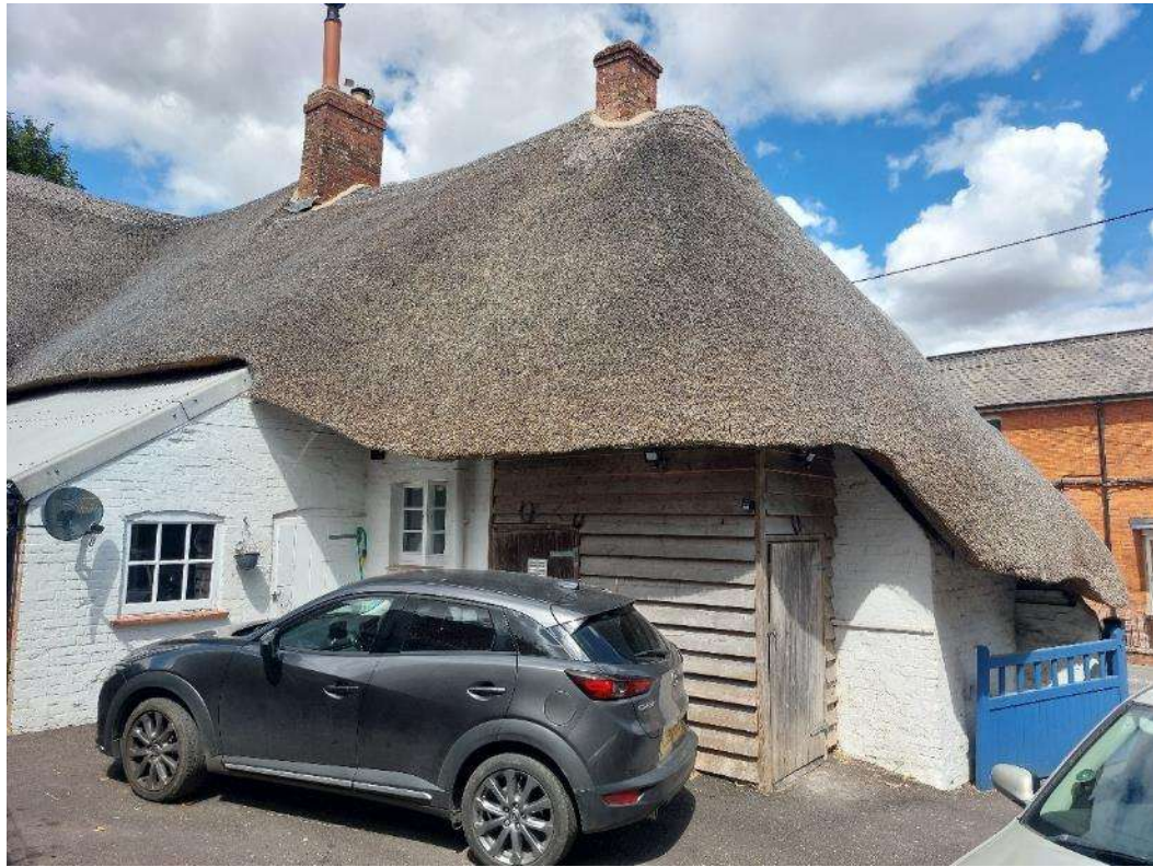
Figure 10 The southern end of the house, rear and south elevations.
