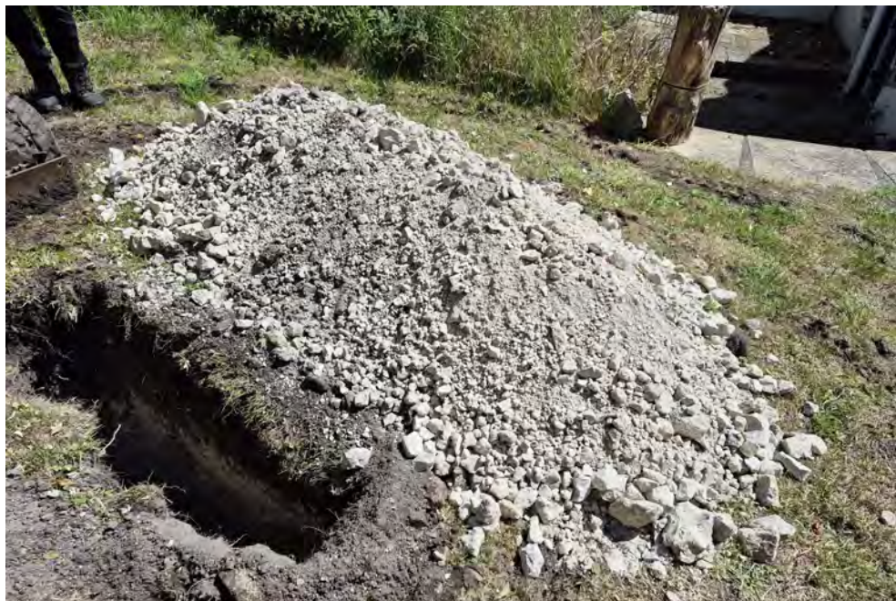
Photo of trial pit SA02 Arising
