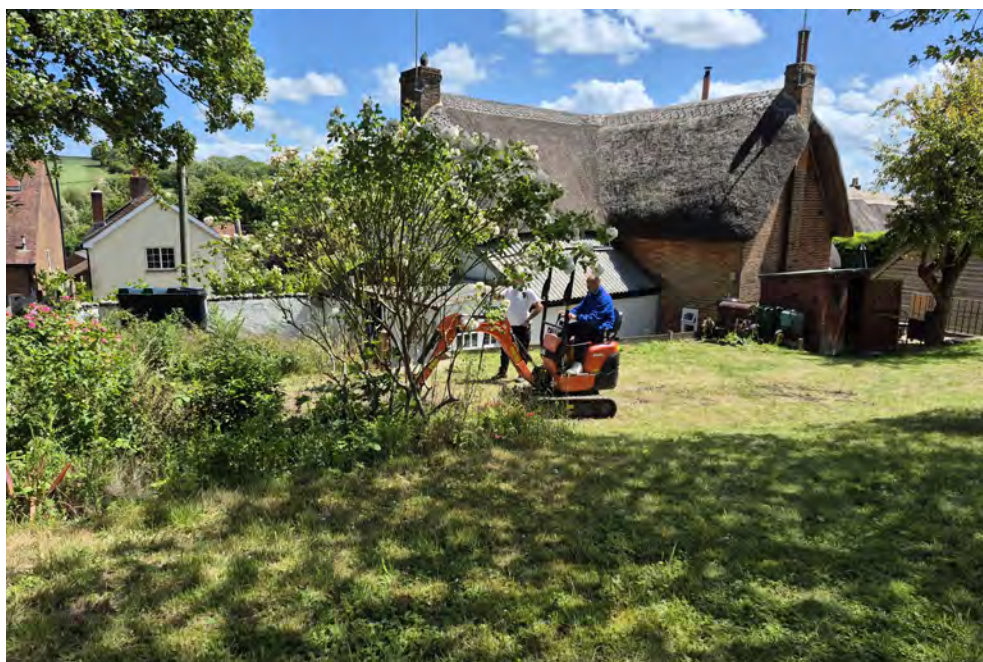
Photo of the investigated area facing southwest
