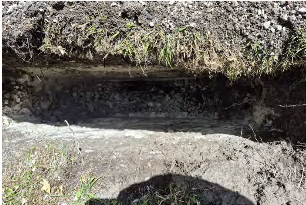
Photo of trial pit SA02
