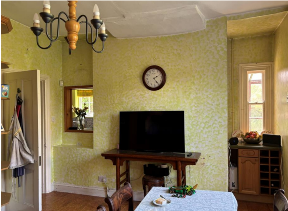
Fig.3 Existing West Kitchen Wall with Existing Opening to Utility and Blocked Up Fireplace.
