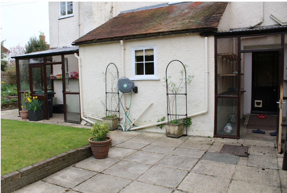
Fig.1 Existing Rear Extensions
