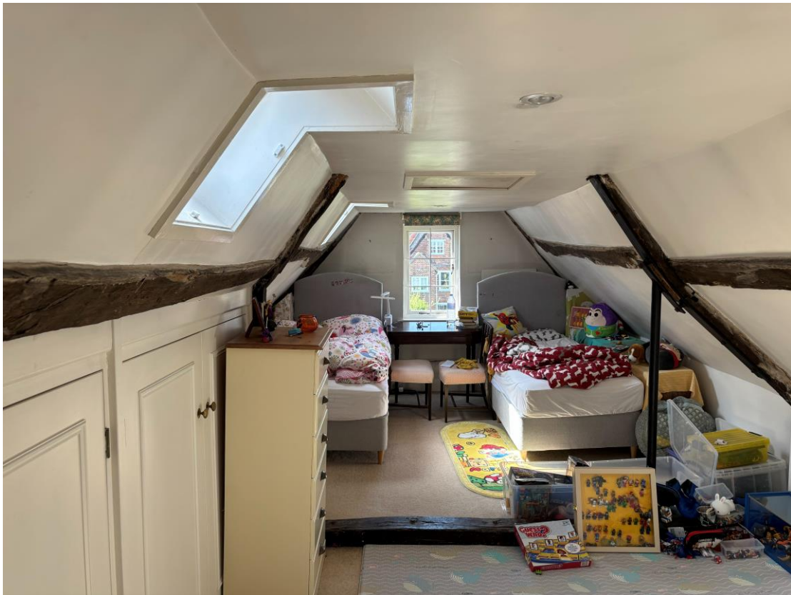
View looking west within Bedroom 5 – modern plasterboard ceiling and rooflights
