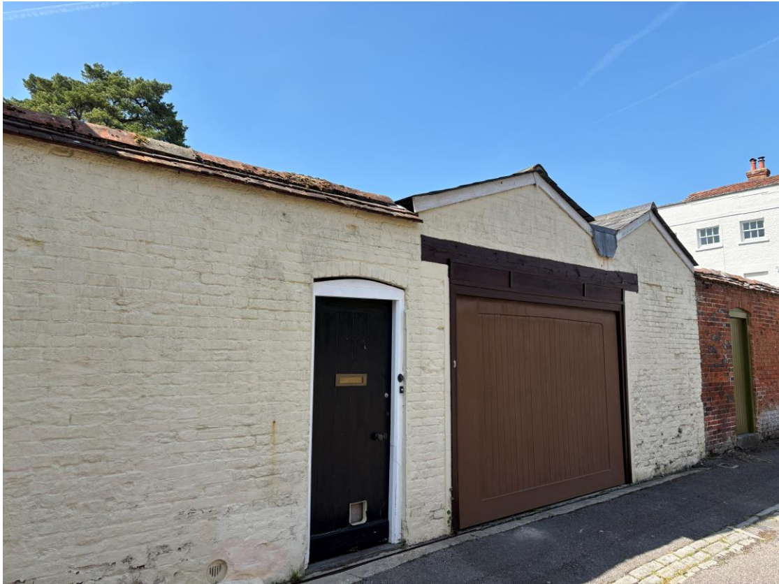
Double gable of the modern buildings cutting through the boundary wall and capping
