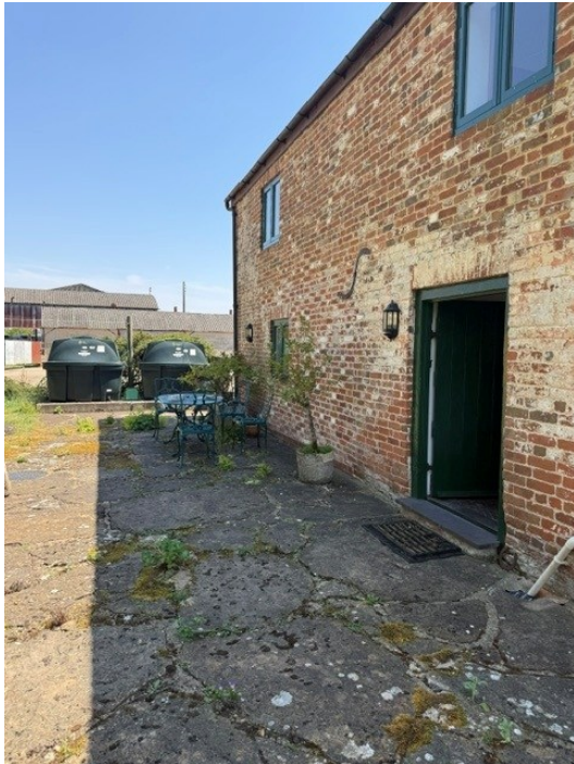
View of rear elevation (North)
