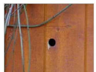
▲ Installation behind wooden panels
