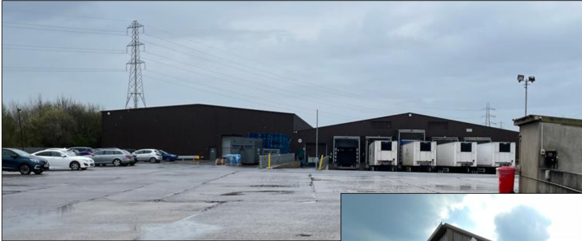
View of existing north elevation of factory building
