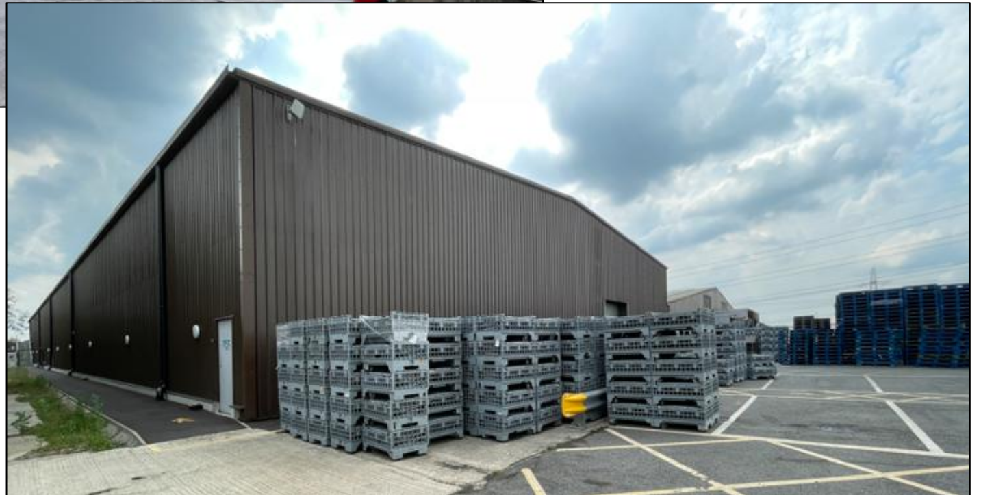
View of existing north elevation of factory building
