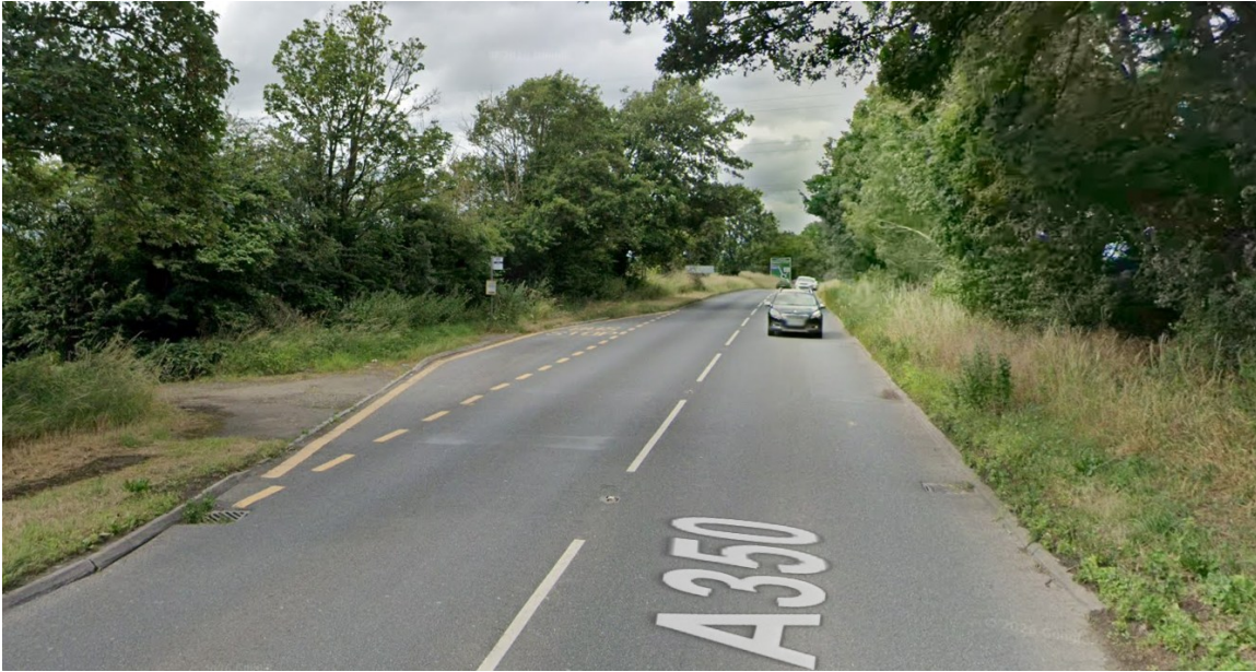
Figure 2 - Current Bus Stop (A350 Northbound)
