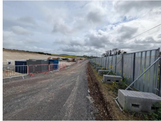
Figure 4.2. Gravel access within the southern extent of the site
