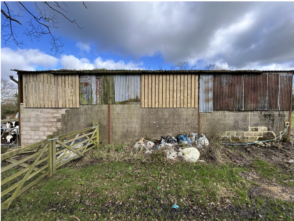
Photos 3 and 4: Photos showing the rear (top) and south western (bottom) elevation. The rear of the building abuts a small stable. The proposals seek to use the land in the foreground of the south western elevation as curtilage for the proposed dwelling.
