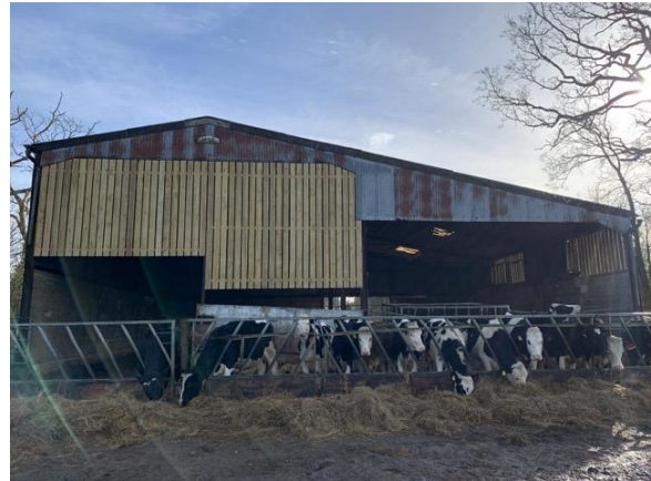
Photo 11 Barn north west elevation
