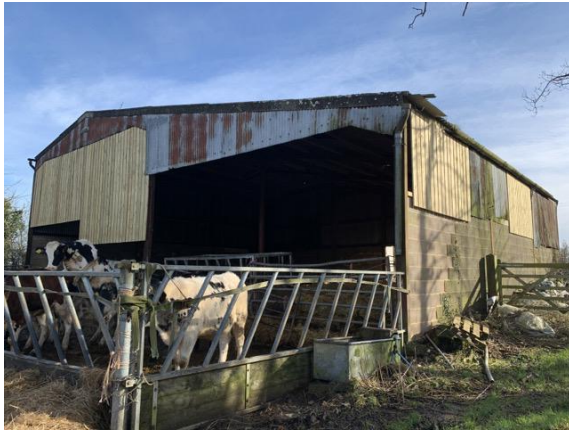
Photo 10 Barn north west elevation
