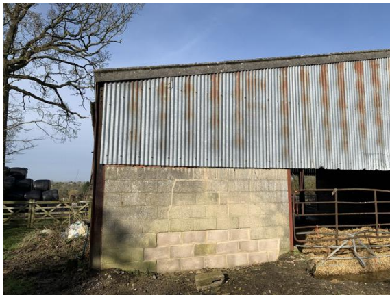
Photo 12 Barn southeast elevation
