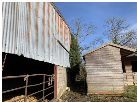
Photo 15 Barn east elevation with adjacent shed outside of red line
