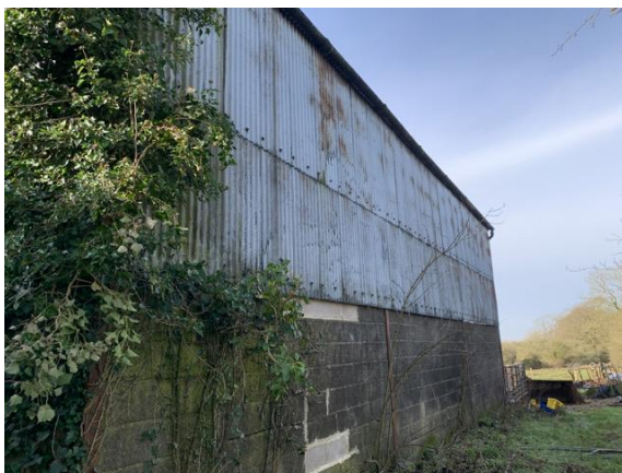
Photo 14 Barn north/northeast elevation
