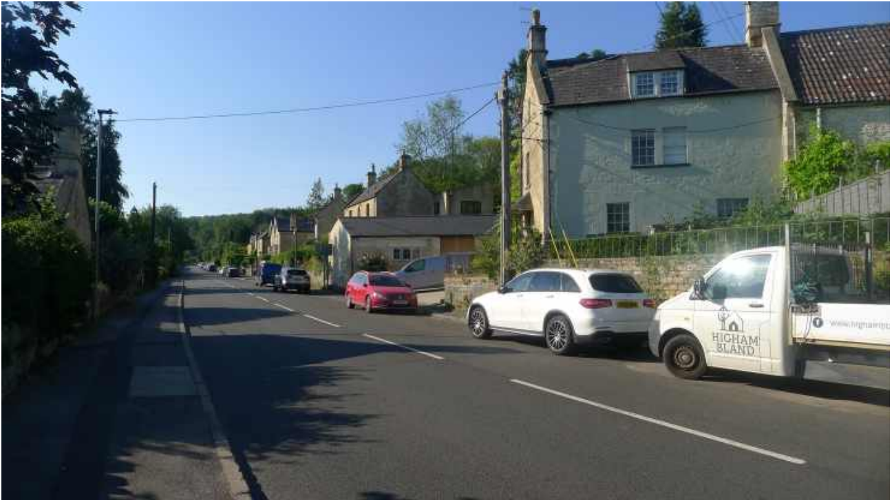
Former Lamb Inn Public House converted to dwelling at Pye Corner (note converted outbuilding beyond (residential)).
