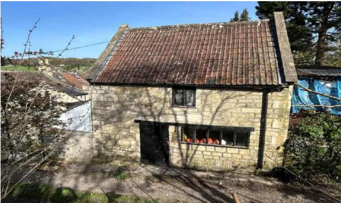
View of Blacksmiths Cottage from garden
