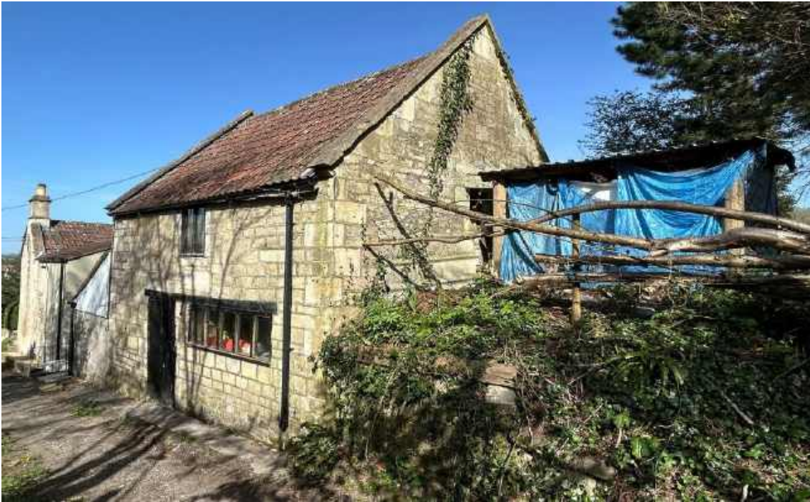
View of Blacksmiths Cottage from byway
