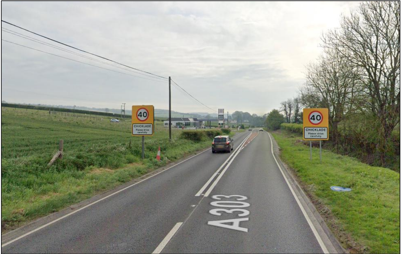
Figure 3-2: A303 (view eastbound)
