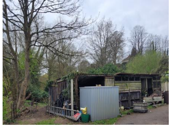
Photo 2: A general view of the site from the north-east.
