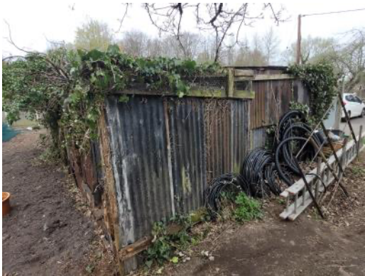
Photo 3: A view of the timber framed outbuilding from the rear.
