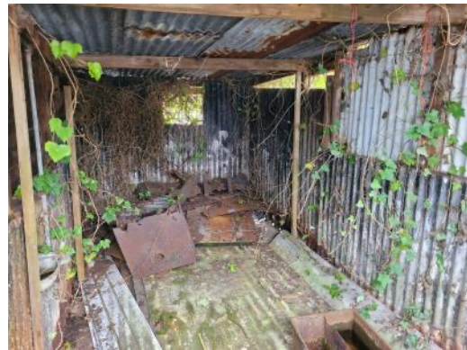
Photo 4: An internal view of the timber framed outbuilding.
