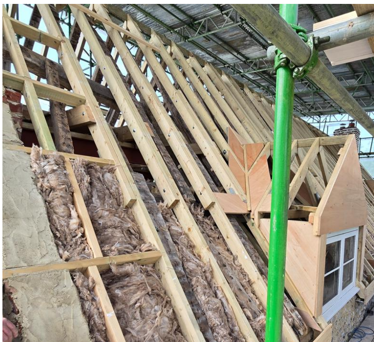
New rafters installed, high level bolted collars bear on the purlins and a new wall plate has been formed, the original roof structure with its lath and plaster linings preserved within.
