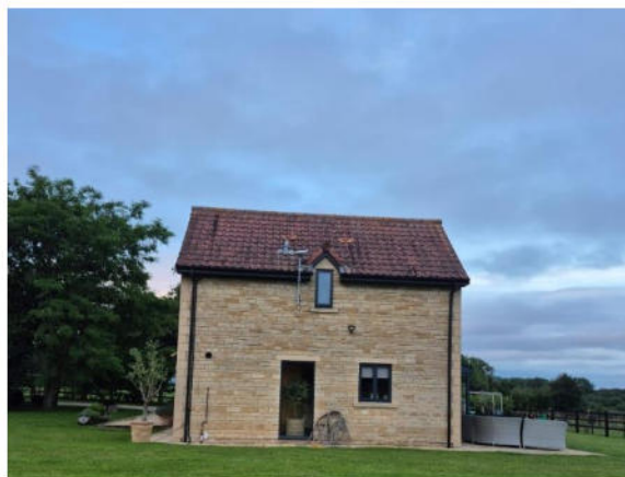
Photo 2 – View of building 1 from the position of surveyor 1.
