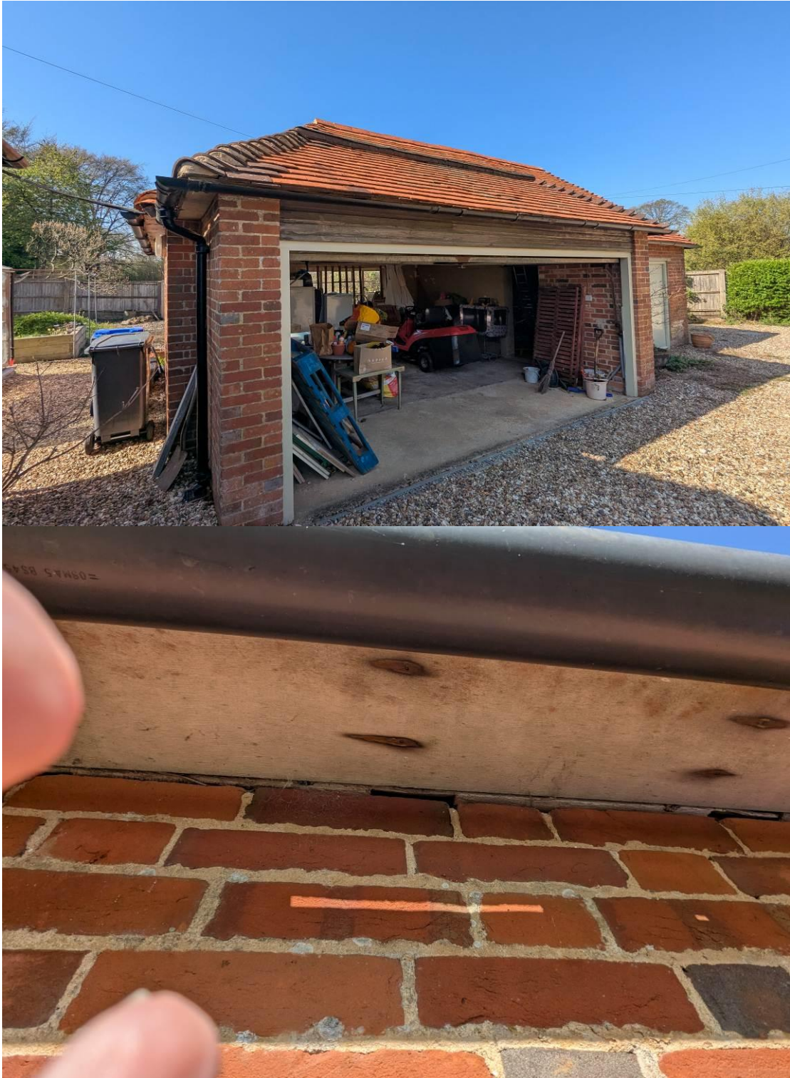
Photo 11/12 The Old Livery, no recorded internal evidence of bat use to date
