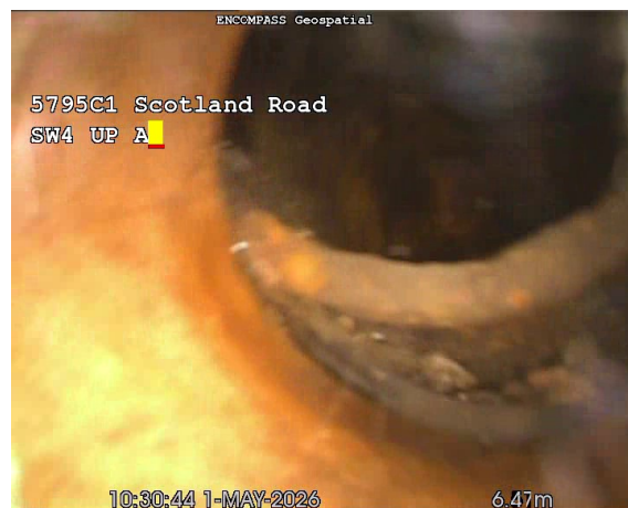
SW5X_4cfb9dfb-1a55-4993-bdf2-4b12c2f311d5_20260511_102019_781.jpg, 00:01:40, 6.47 m Joint displaced, large
