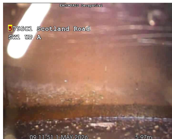
SW1 UP AX_45194fd8-d74b-4e0c-92ef-a9e5812af181_20260511_10044 4_741.jpg, 00:00:45, 5.97 m Finish node, gully, reference: GY1
