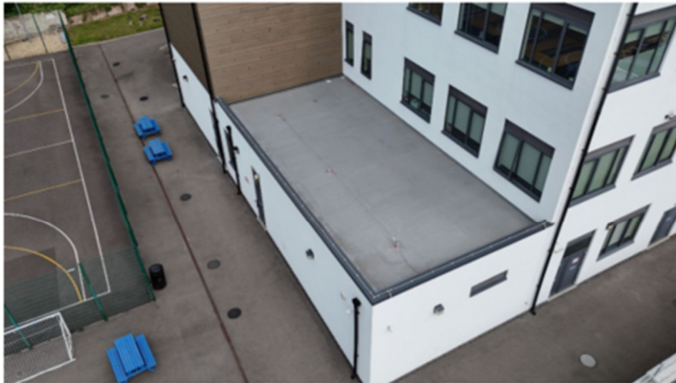
Photo 5 – Single storey, south east corner of existing building (location of proposed vertical extension)
