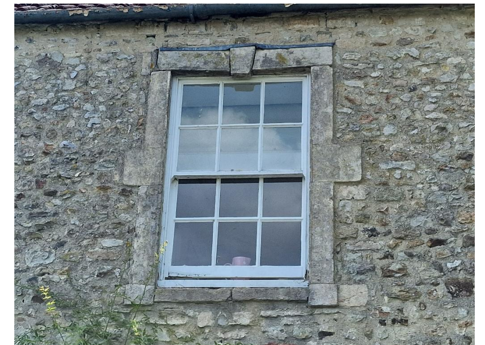
Figure 6: Main elevation boxed sliding sash windows.
