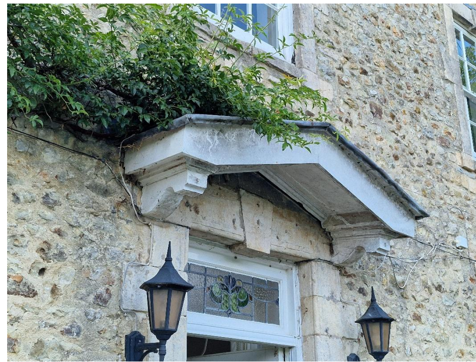
Figure 8: Timber and lead front door cover
