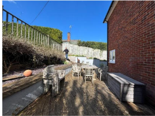
Rear of house for new extension
