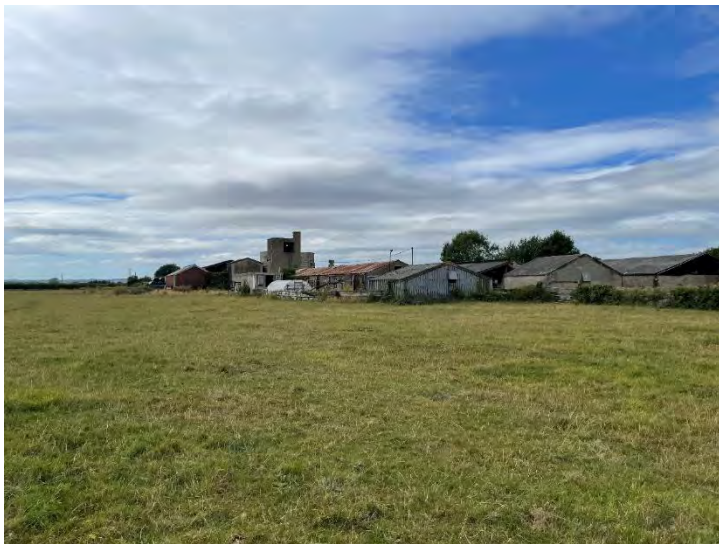
Plate 24: Complex of farm buildings, including WWII structures, as seen from the southwest.
