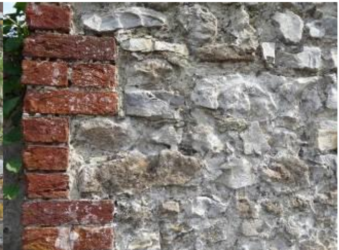
East side front jamb
