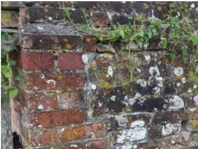
West side rear jamb
