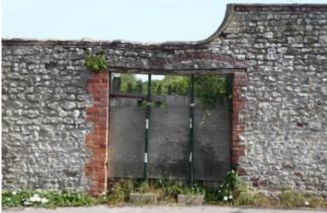
Gateway from the front (road)
