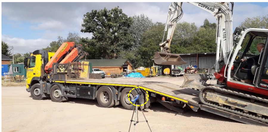
3: Example of noise measurement of plant movement
