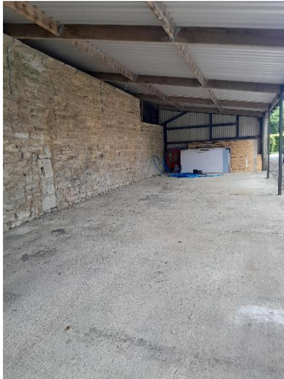
Photo 6. Inside B2 looking towards B1 (west)
