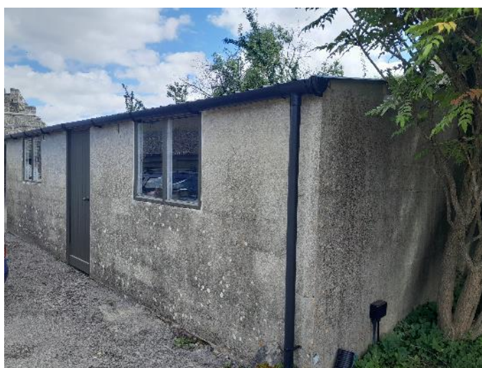
Photo 1. B1 northern and western elevations
