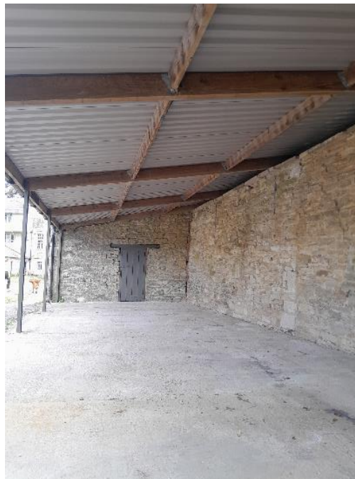
Photo 5. Inside B2 looking east
