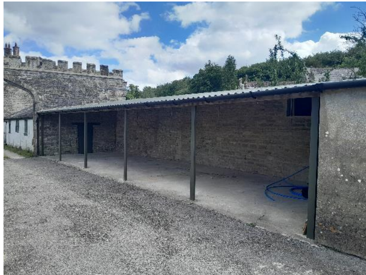
Photo 4. Northern elevation of B2
