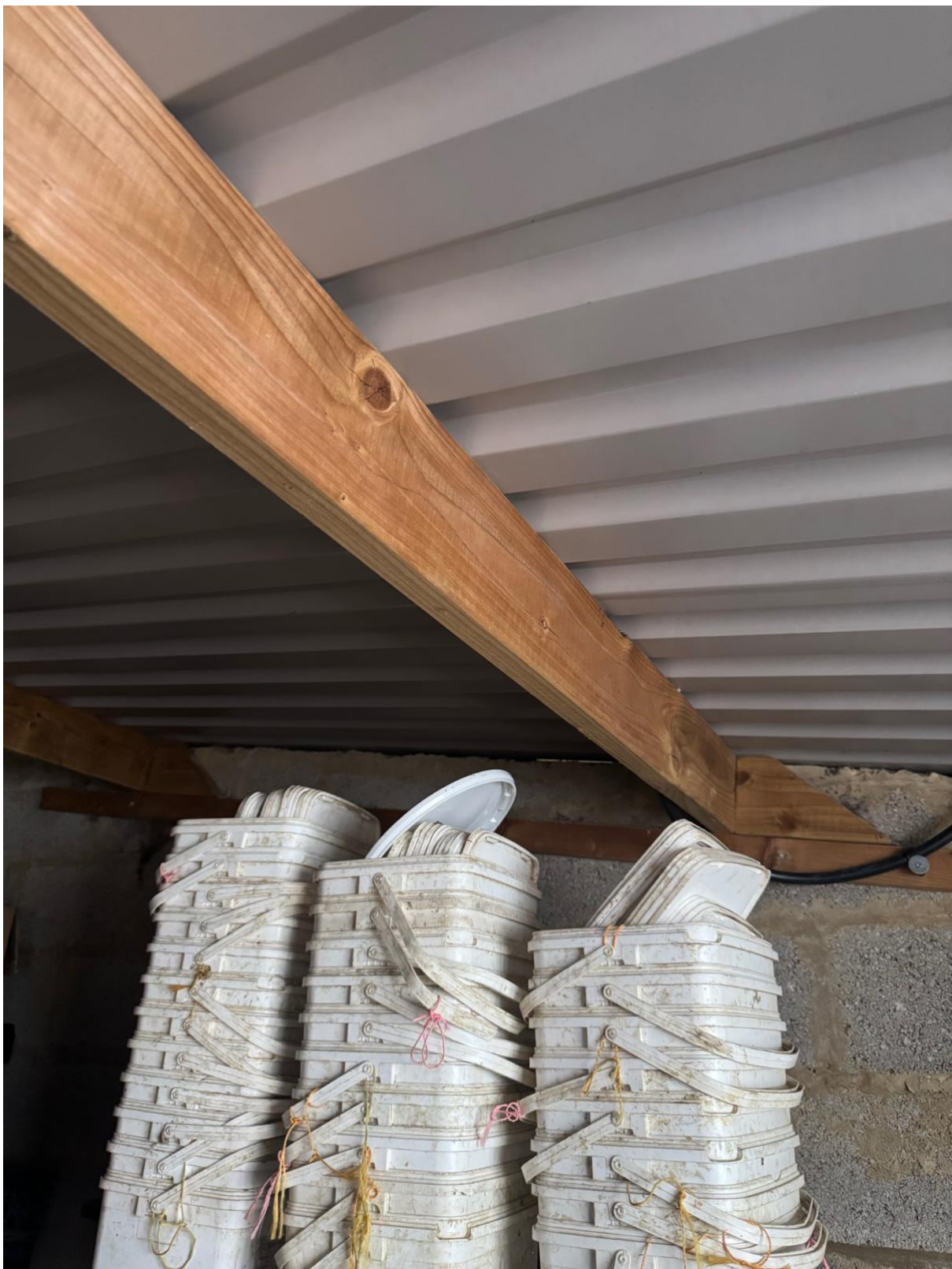
Figure 15: Sawn softwood timber principal rafters
