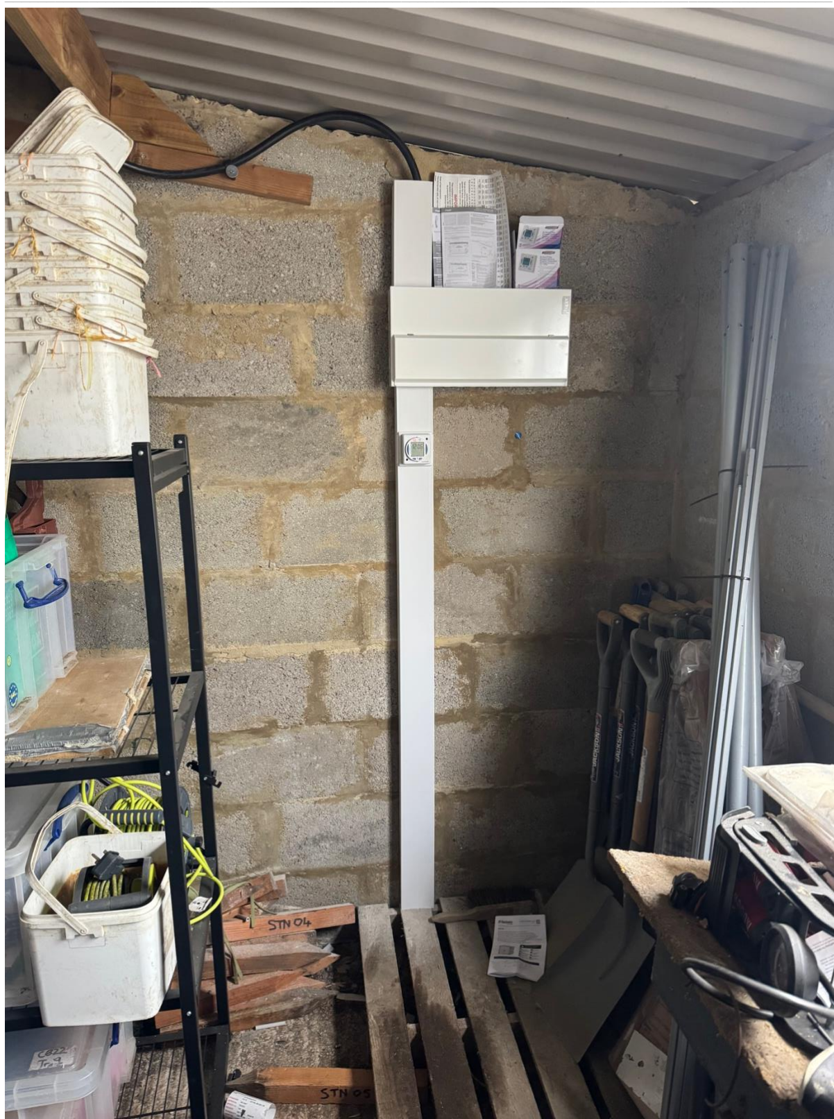
Figure 13: North-west wall (internal) of store
