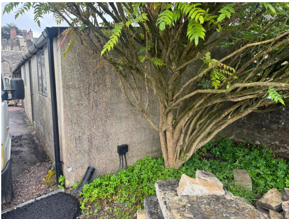
Figure 9: The store on the site and the open lean-to beyond
