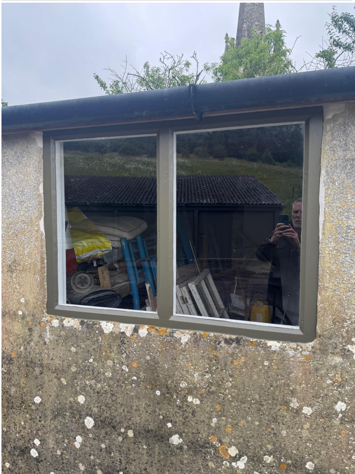
Figure 11: One of two, two-light windows to north-east elevation
