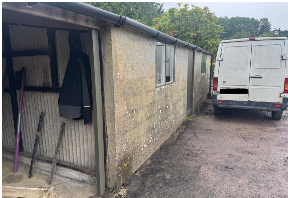
Figure 7: The enclosed section of the building on the site (proposed for demolition)
