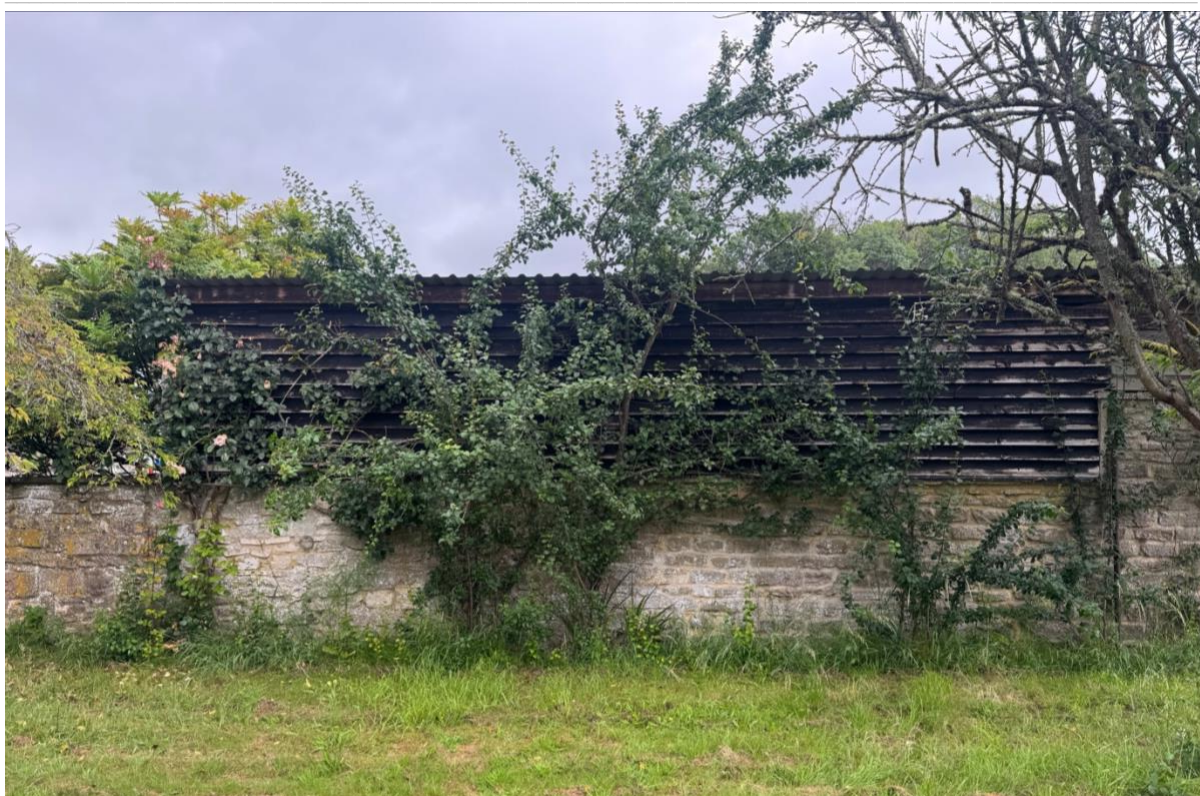
Figure 8: Boundary wall forming the south-west elevation of the store (the site)
