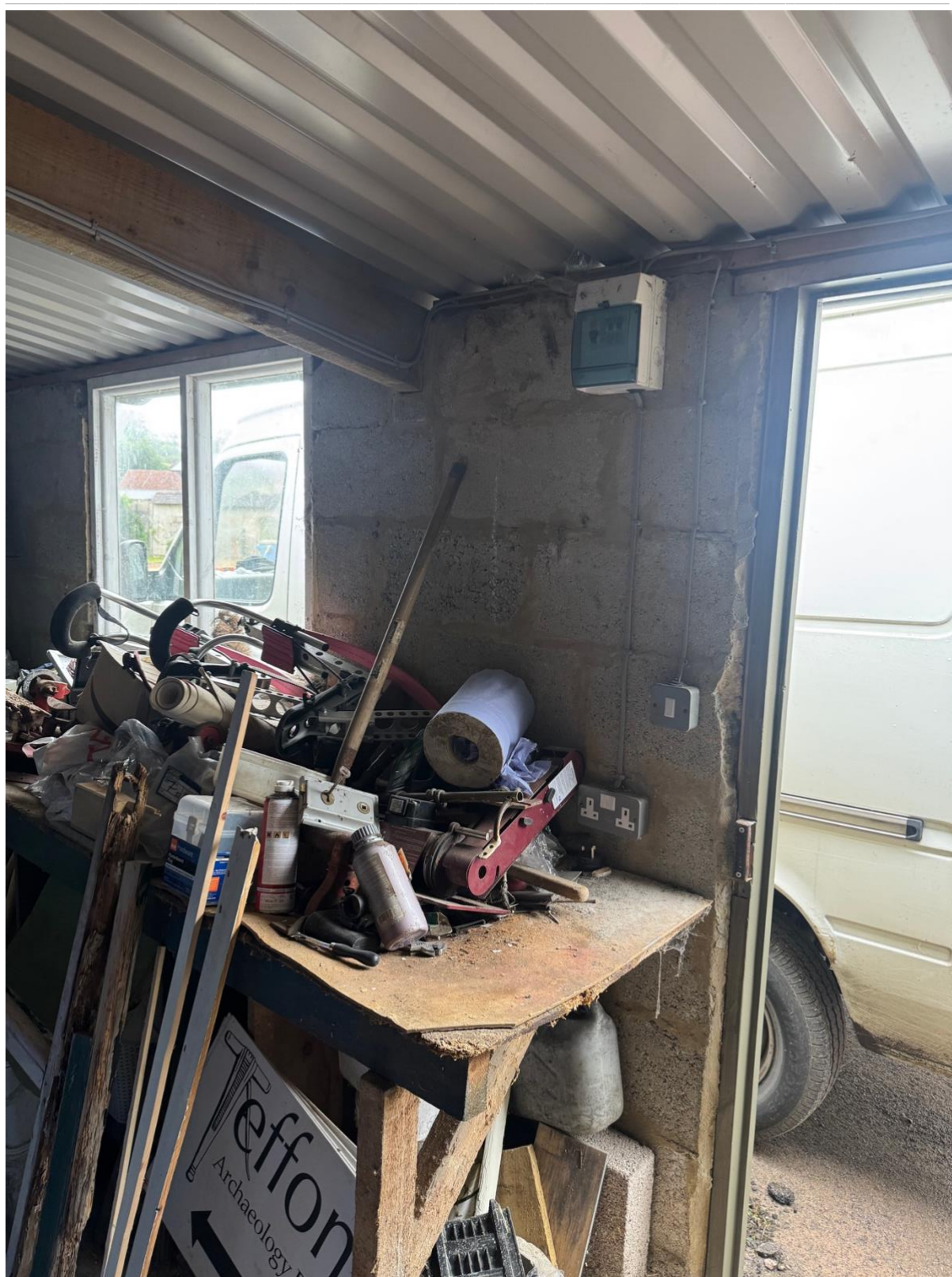
Figure 10: Blockwork to the store elevations (seen to north-east and north-west elevations)
