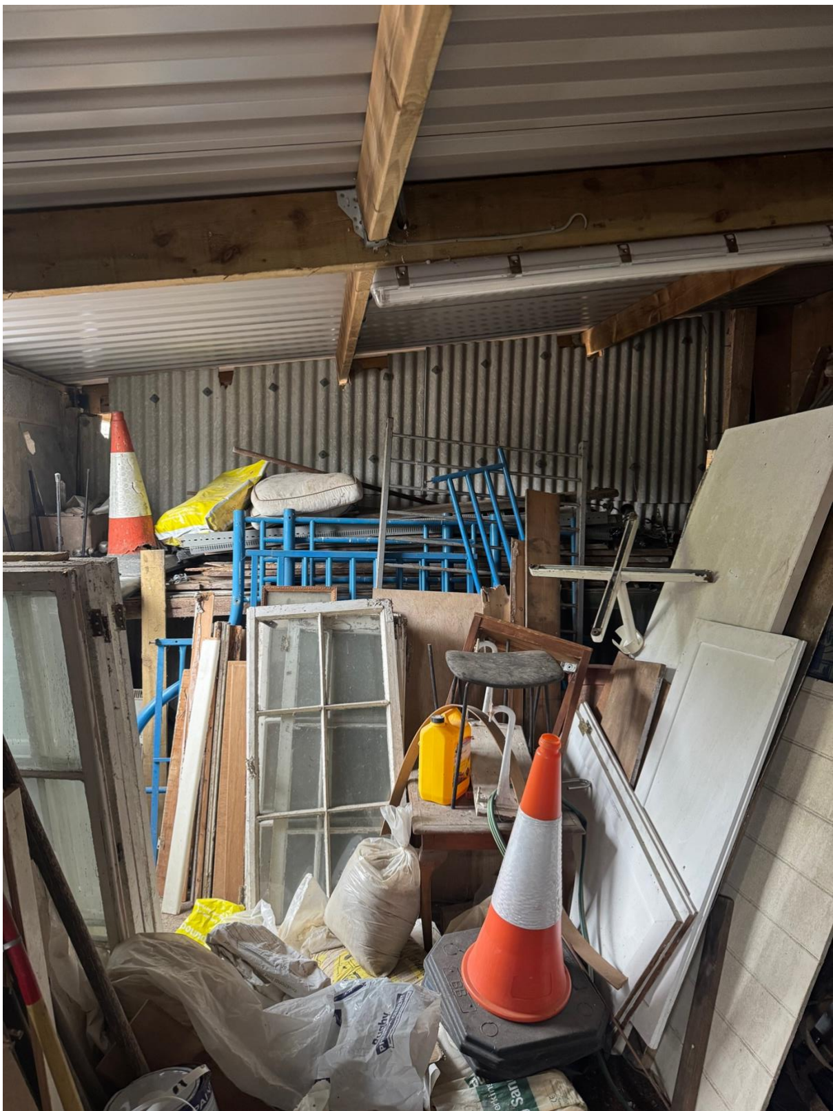
Figure 14: Modern roof structure of store
