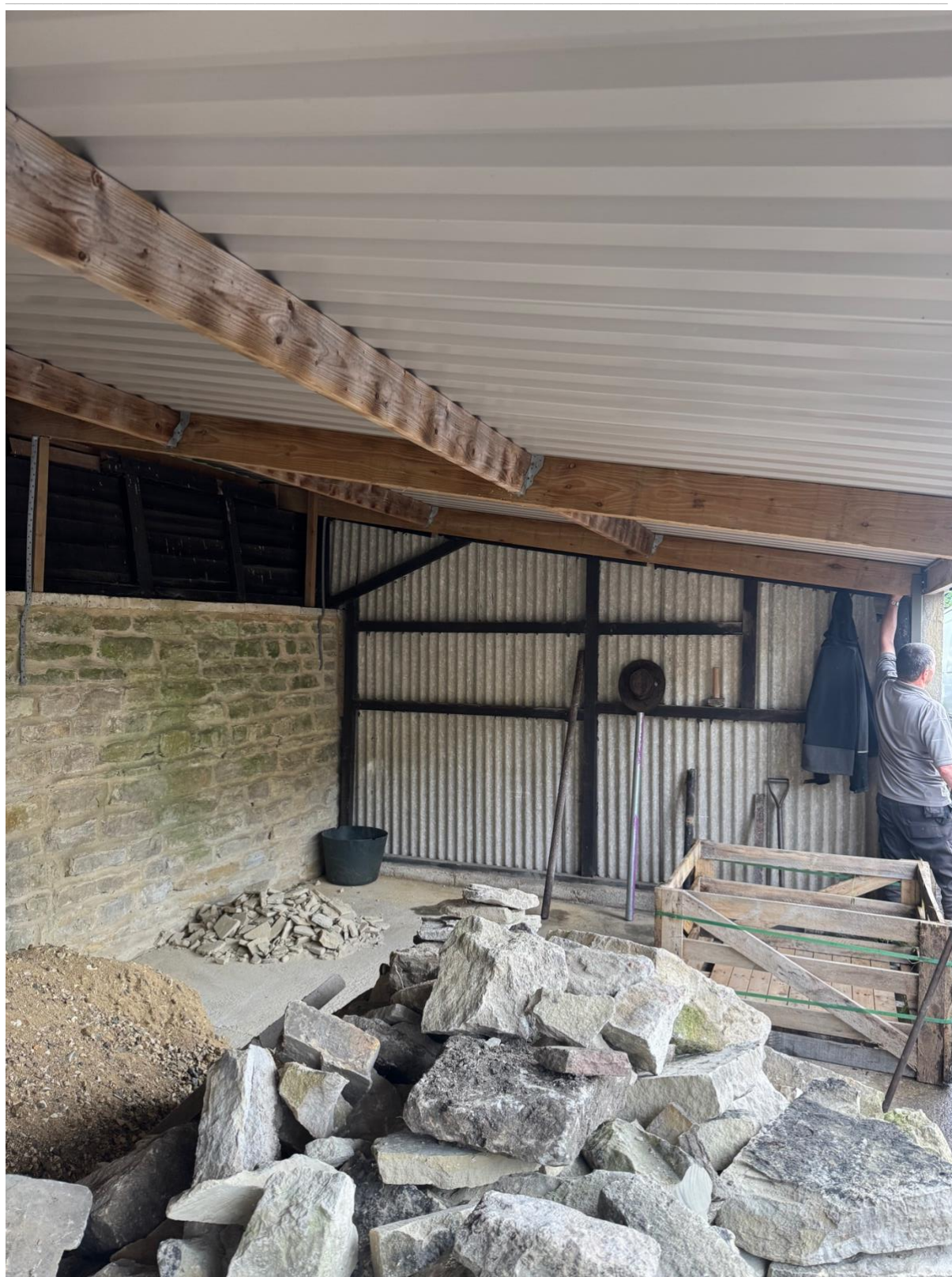
Figure 12: The south-east elevation of the store
