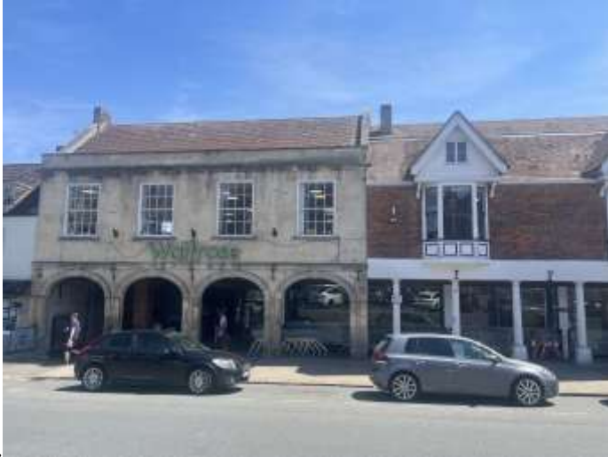
Front façade of Waitrose store
