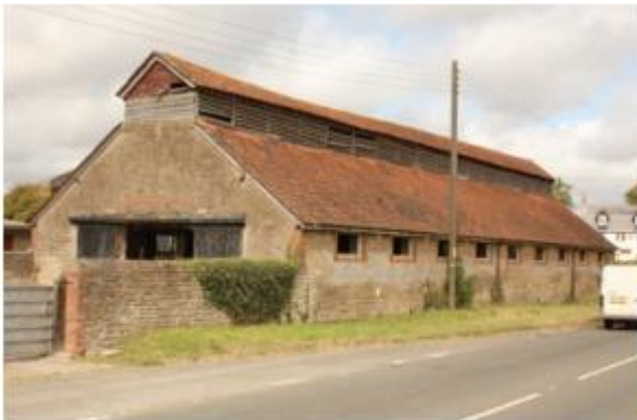
A late 19th century covered yard building with a typical vented ridge and numerous window openings. Photo © Bob Edwards
