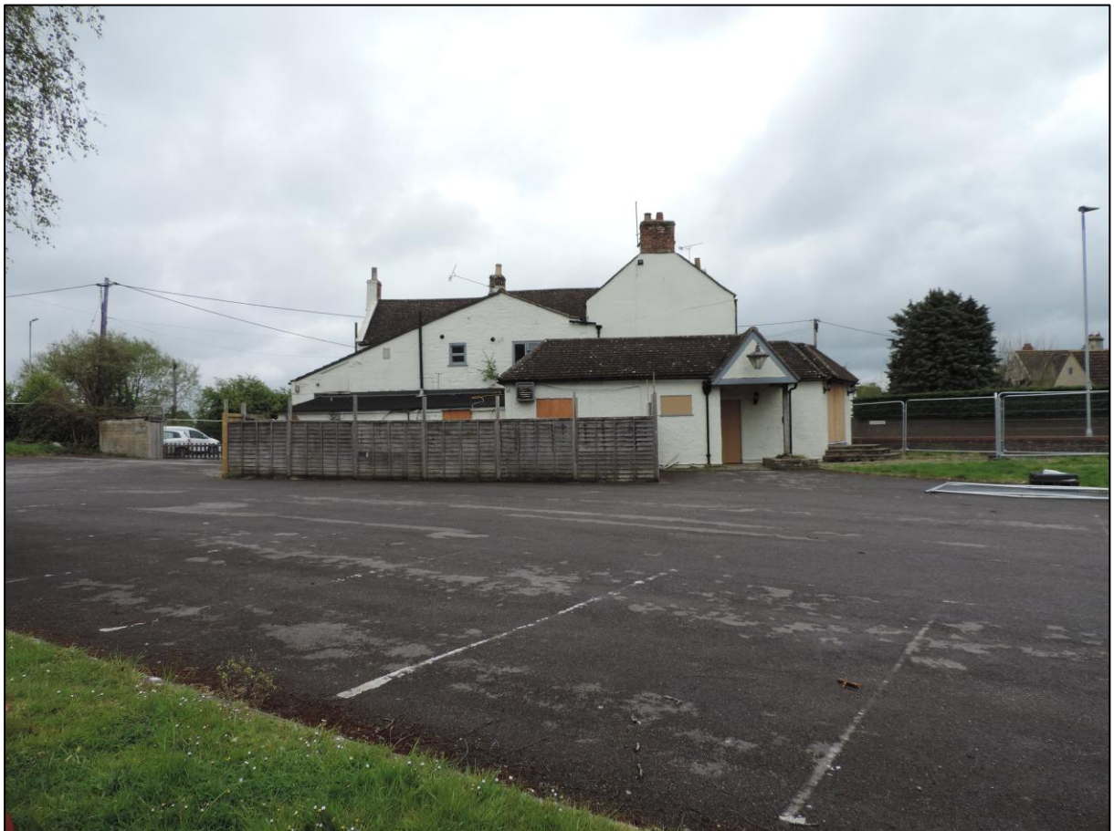
Photo 5 West elevation of the Kings Arms Public House.
