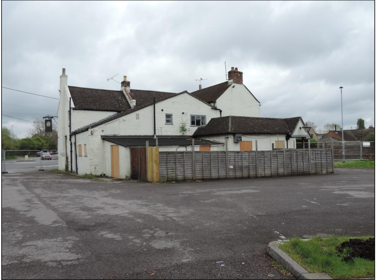
Photo 4 South facing elevation of the Kings Arms Public House with 20 th century single storey extension.
