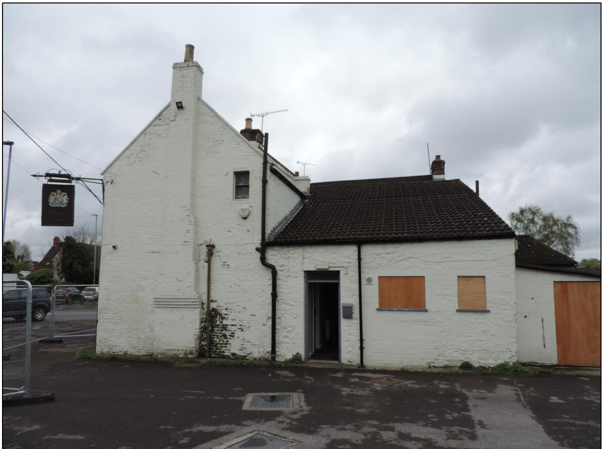
Photo 3 North facing elevation of the Kings Arms Public House from the car park.
