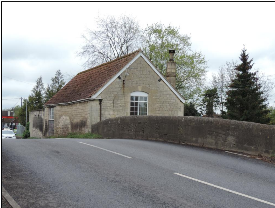
Photo 9 Southeast facing view of Wharhouse No. 2 Marsh Road from the Kennet and Avon Canal Bridge.
