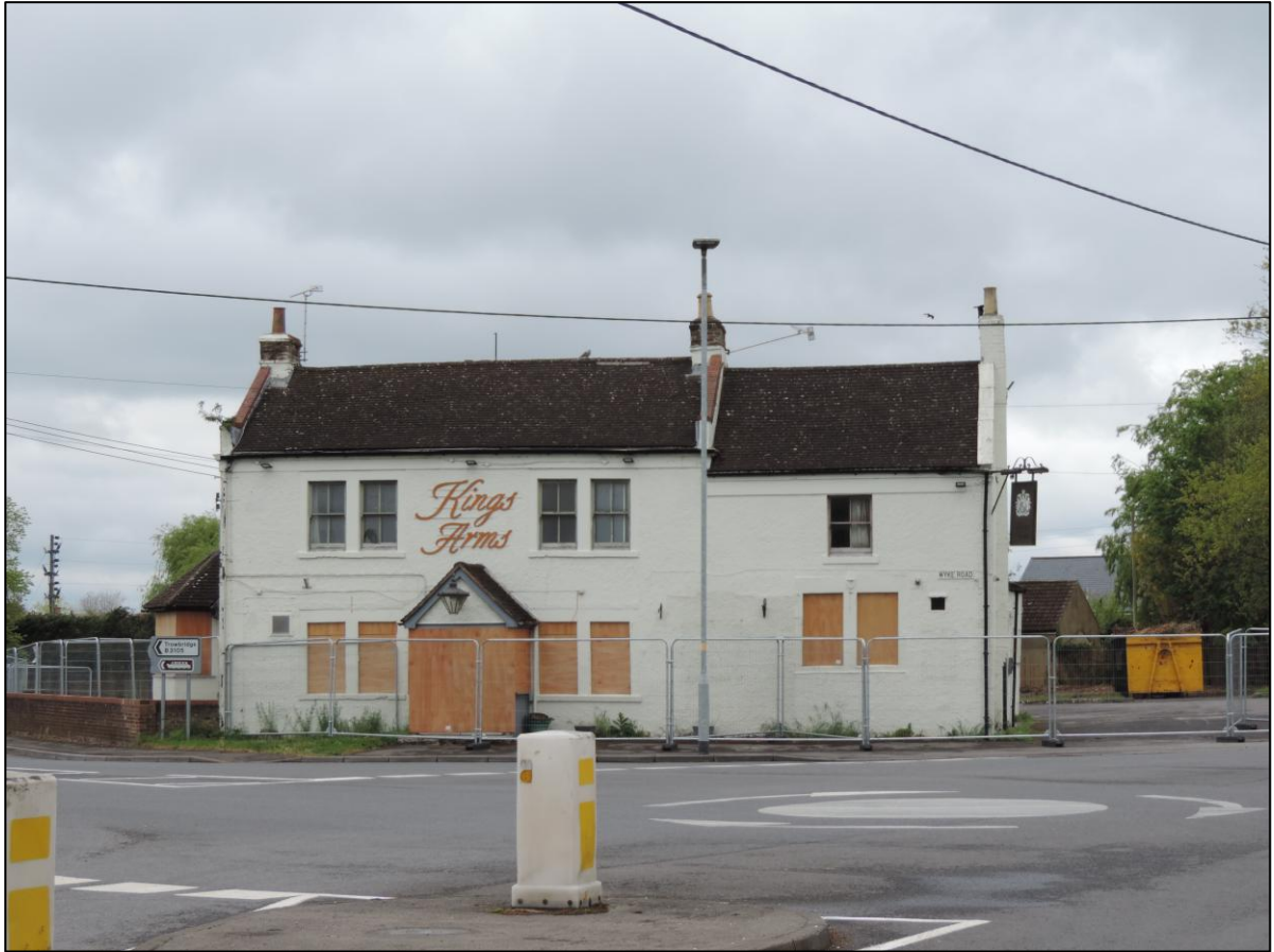
Photo 2 West facing view of the principal elevation of the Grade II listed Kings Arms Public House, no. 79 Wyke Road.
