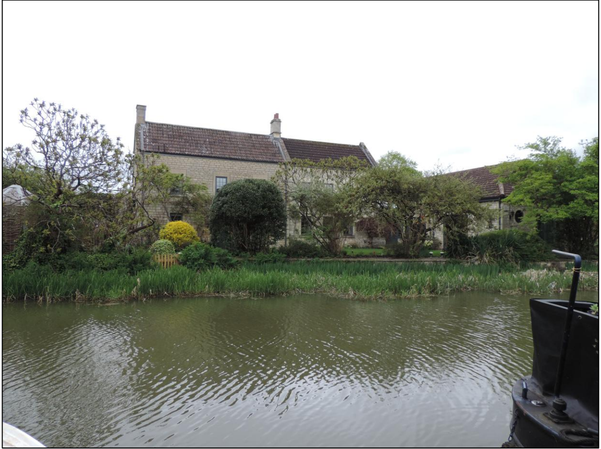
Photo 10 ESE facing view of the principal elevation of Kennet Cottage from the towpath. The rear roofline is visible from the Project Site.
