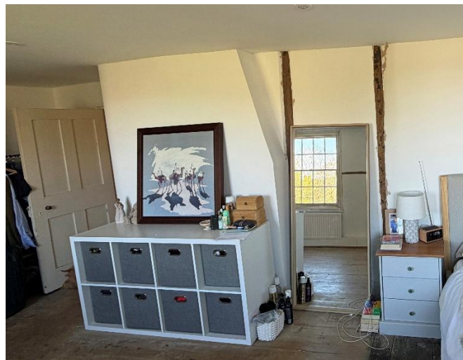
Fig.104 Two studs, south-east partition
