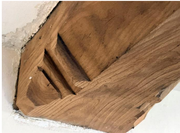
Fig.34 Double roll and concave stop
