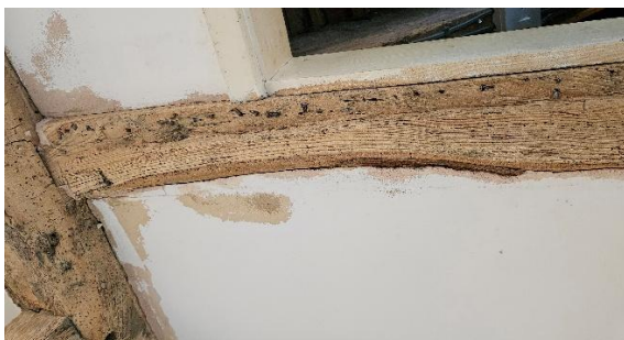
Fig.69 Ceiling beam with nail evidence of former partition
