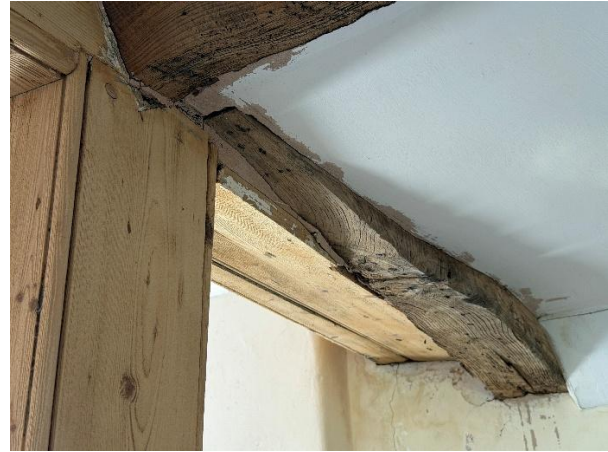
Fig.68 Tapering, nailed splint
