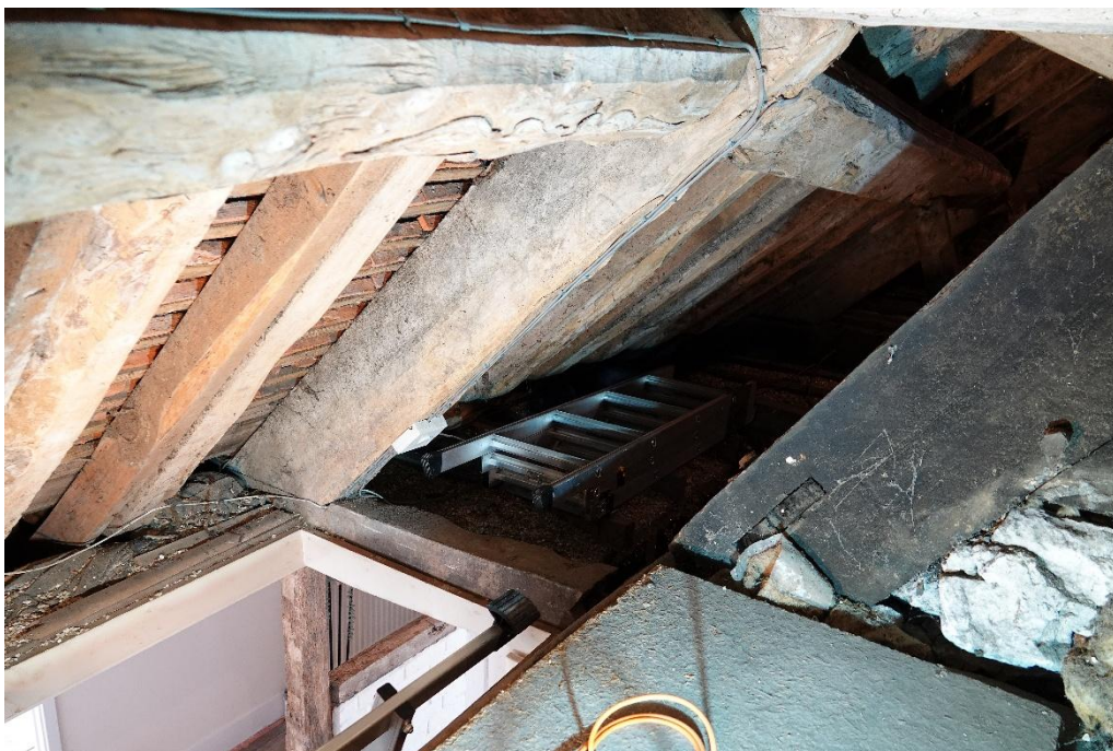
Fig.130 This view shows to the SE of the stack shows the blackened principal of T2 to the right, and the unblackened principal of T2A, with its lower purlin tier
