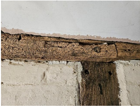
Fig.97 Wallplate scarf joint
