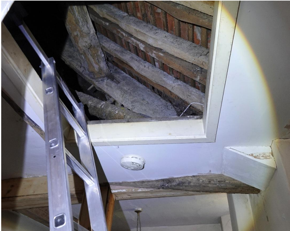
Fig.135 Truss T3, looking up through the loft hatch. The principal and its tiebeam, and a purlin, can be seen
