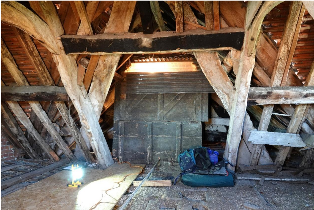
Fig.151 The crosswing looking SW into the hall and cross-passage roof. The principal rafters of T4 and T5 are seen central in this photograph, with the valley boards immediately behind them
