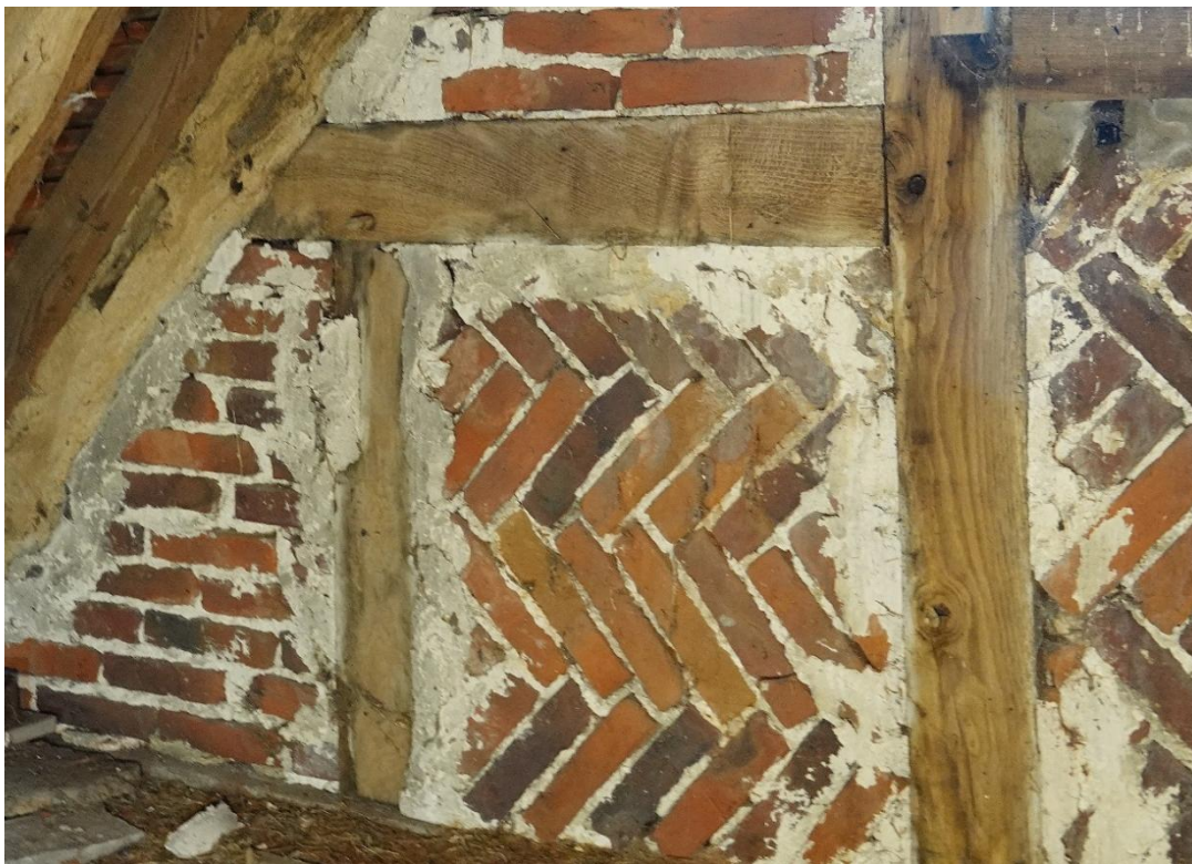
Fig.148 Detail of the timber-framing of the front (NW) gable
