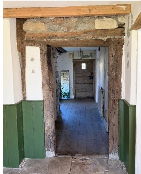
Fig.29 Short length of beam with 3 joist pockets in situ, now embedded within the stonework of a later fireplace
