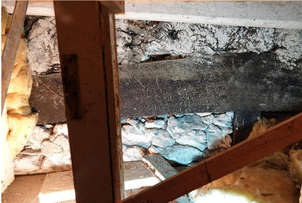
Fig.121 The collar of T2 seen from the NE, with a pronounced crank to its upper face, and central stud. Above the collar is limewashed infill with some soot particles; the stone stack has been underbuilt beneath
