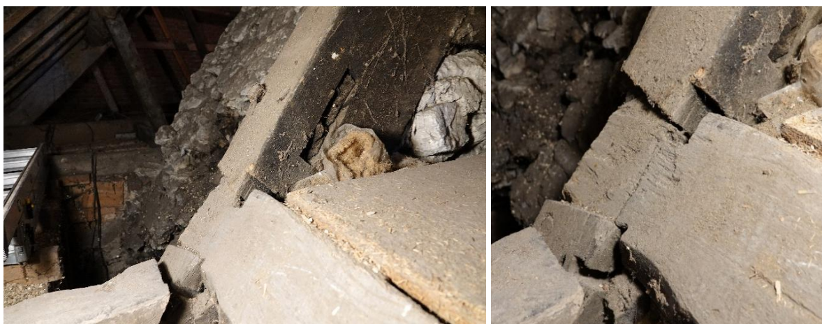
Figs.124 & 125 A short purlin-like timber set immediately below the lower purlin of T2. Note the dovetail joint
