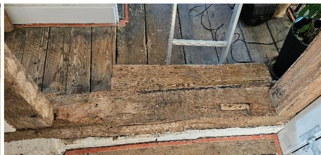
Fig.69 Ceiling beam with nail evidence of former partition
