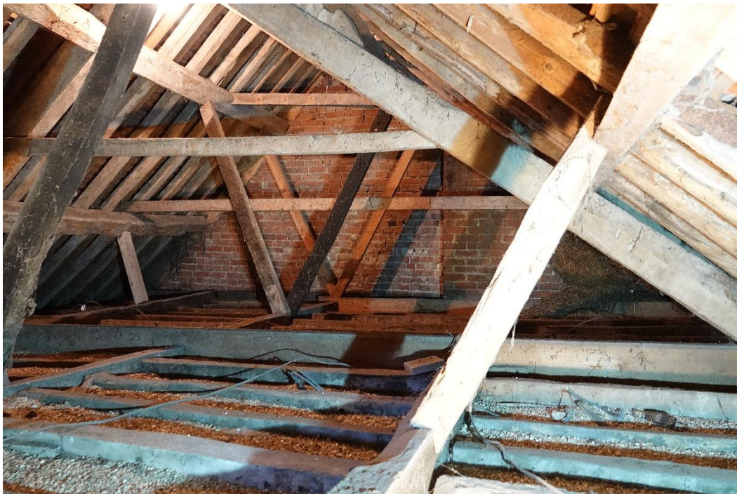
Fig.132 The SW end of the hall roof. To the left the principal and purlins of T1 can just be glimpsed, but the rafters, struts and props are all later; note the blackened common rafter re-used as a prop
