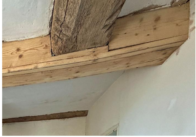
Fig.59 Straight joint in floorboards Fig.60 Elm beam stop-chamfered on both faces
