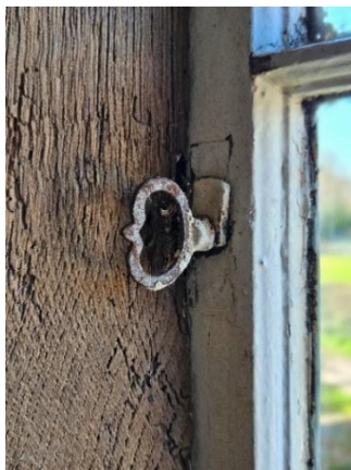
Fig.85 Turnbuckle catch
