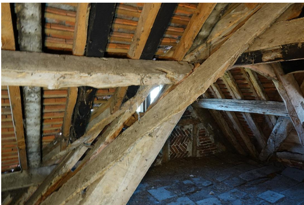
Fig.136 The purlin from T2A running onto the outer face of T5
