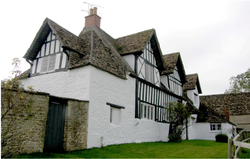
Fig.11 Catridge Farm, Lacock; a later 16 th century farmhouse and semi-basement dairy (in foreground). This yeoman farmhouse also has timber-framing built off a high plinth. Wiltshire Buildings Record has recorded numerous such examples, including farmhouses and cottages in the Devizes area
