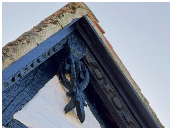
Fig.20 Open pendant at apex of gable
