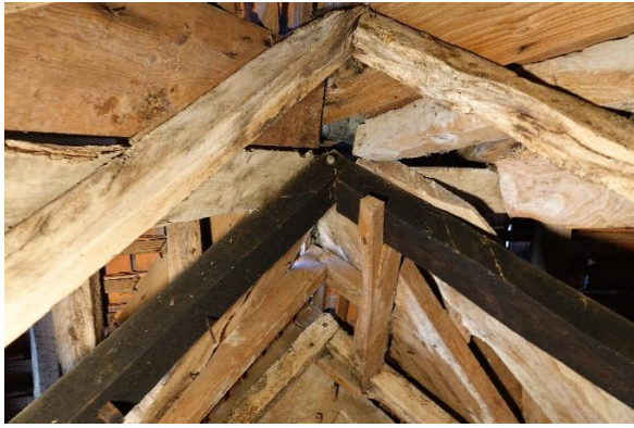
(left) Fig. 139 A re-used rafter pair in the crosswing roof. (Right) Fig. 140 Gouge marks on T5
