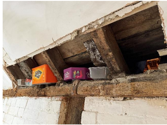
Fig.98 Extension has machine-sawn rafters, supported on the old wallplate
