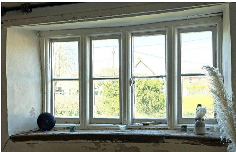
Fig.39 4-light ovolo-moulded mullioned window
