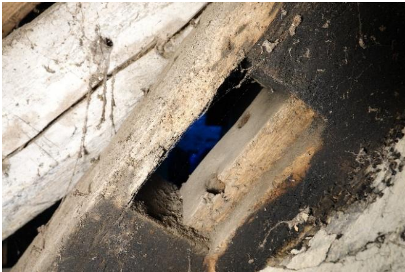
Fig.123 T2, the vacant mortise for the butt purlins, upper tier, each single-pegged
