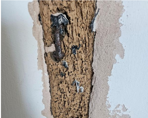
Fig.105 Iron nail, south-west stud
