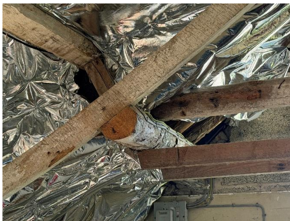
Fig.155 Altered roof truss with modern strutting replacing earlier struts
