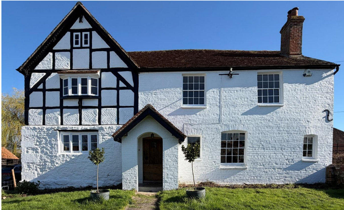
Fig.18 Front (north-west) elevation
