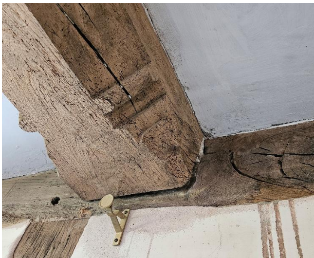
Fig. 75 South-east beam joint; north-east wallplate chamfer respects the beam
