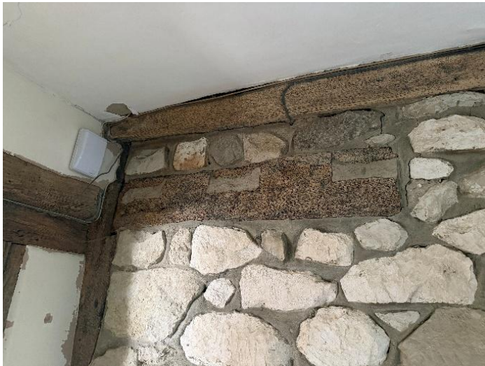
Fig.29 Short length of beam with 3 joist pockets in situ, now embedded within the stonework of a later fireplace
