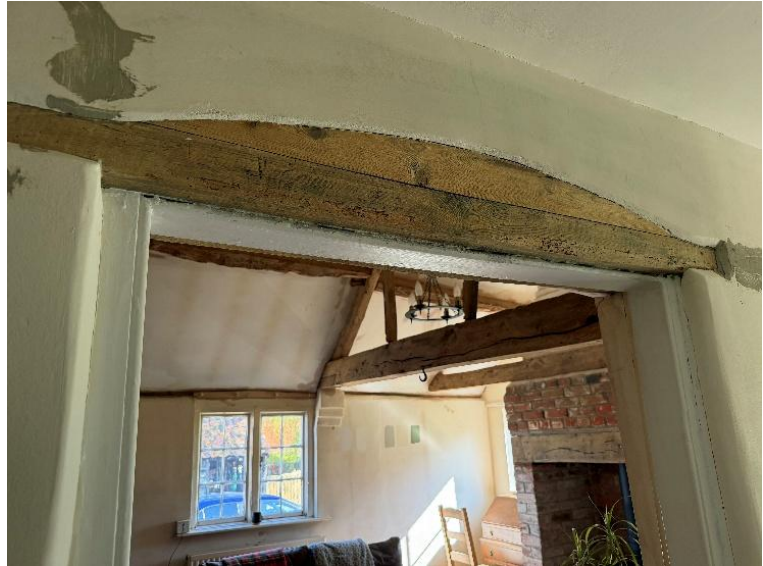
Fig.45 Segmental head to back kitchen entrance
