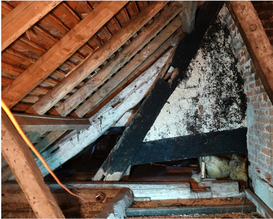
Fig.116 Truss T2 from the SW, showing the cranking of its collar; and the principal and tiebeam of T2A
