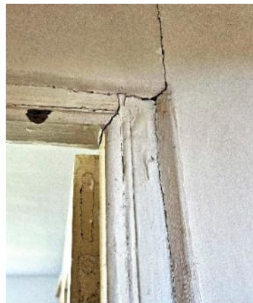
Fig.112 Bead & torus-moulded door architrave, landing face
