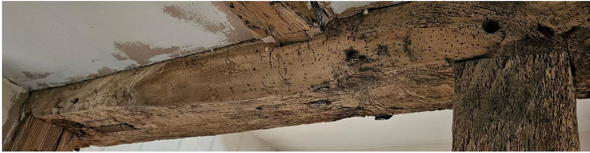
Fig.71 Redundant mortise for former stud in wallplate soffit. Chamfer with runout stops could indicate a former opening.
