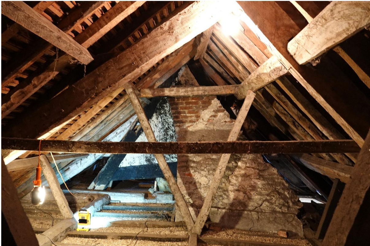
Fig.115 A general view of T2 from the SW. In this view the smoke-blackened truss T2 is seen behind the stack; the NW principal of T2A can be seen to its left. Immediately in front of the camera is T1
