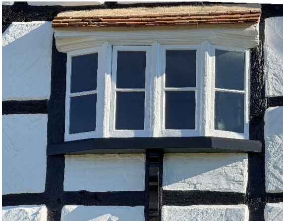
Fig.19 First floor oriel window
