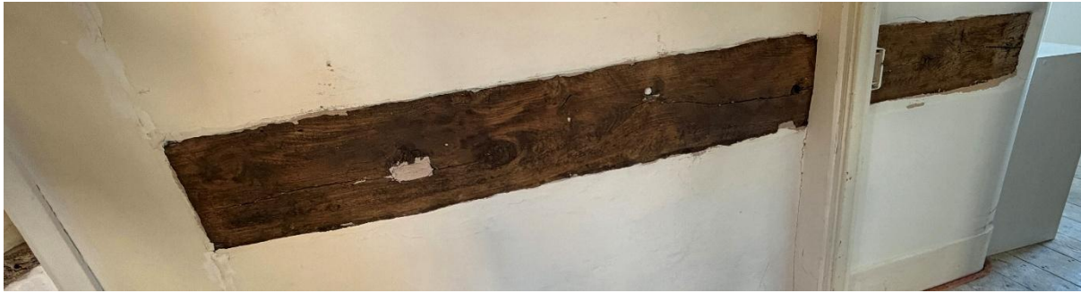
Fig.66 Tie-beam embedded in stack wall
