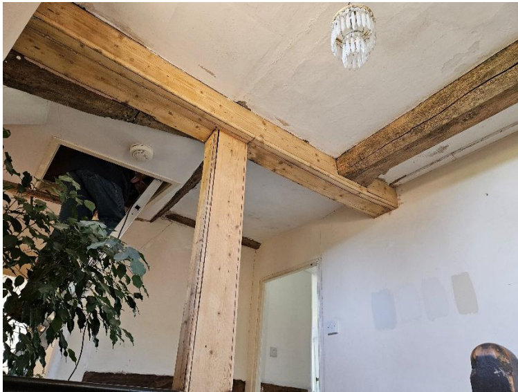
Fig.57 Looking west; softwood beam at junction of two distinct areas
