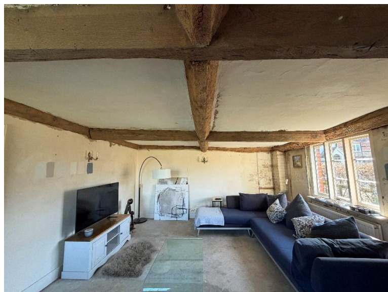
Fig.56 View to rear of room
