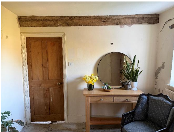
Fig.27 Modern partition to living room (G9). The visible beam butted against the former suggested smoke bay
