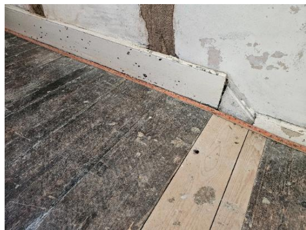
Fig.89 Changes in floor and skirting at location of former partition; bead skirting to left
