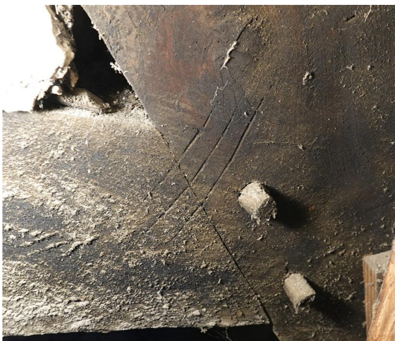
Fig.126 Carpenters' mark on T2
