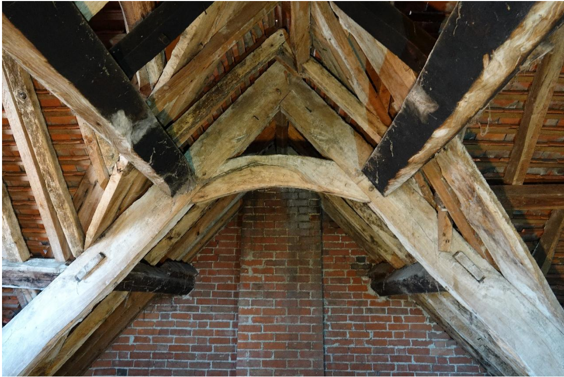
Fig.137 Truss T4 looking SE to the brick rear wall
