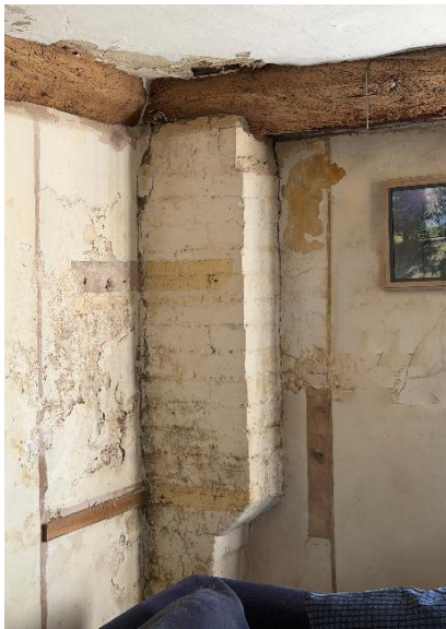
Fig.55 Brick pier supporting ceiling timbers
