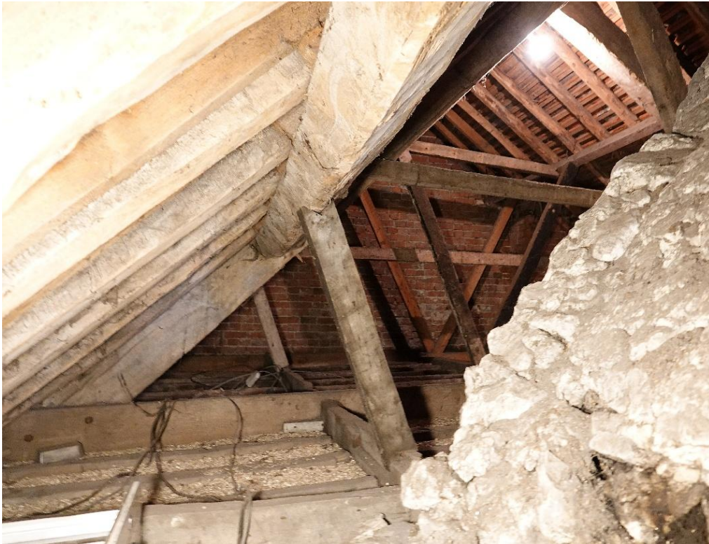
Fig.129 Truss T1, looking SW. One principal rafter can be seen, bolted to a replacement tiebeam, with a lower purlin running into it, now propped
