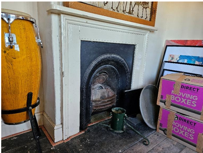
Fig.81 Cast iron arched register grate
