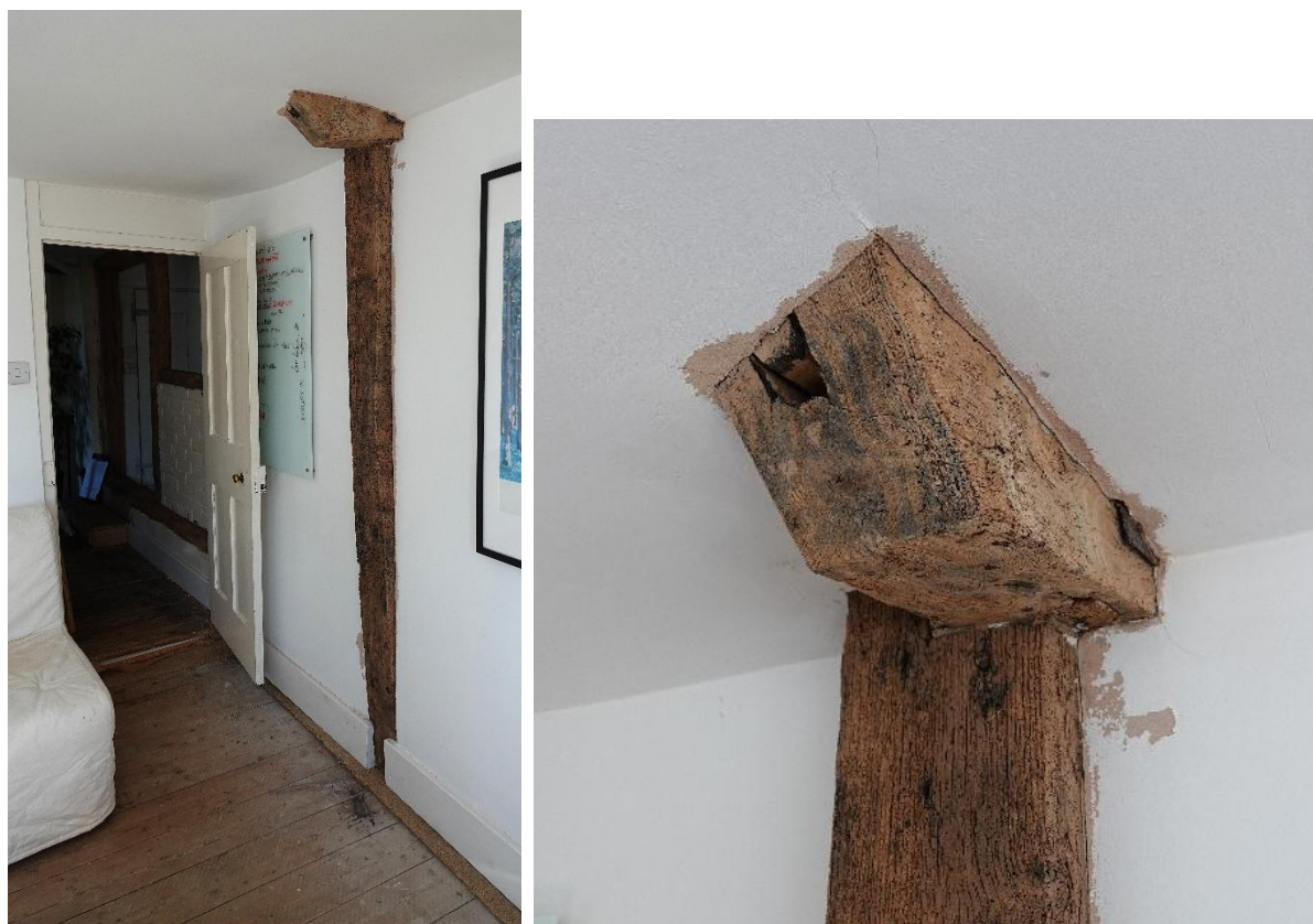
Figs. 127 & 128 The post and sawn-through tiebeam of T1 at first-floor level
