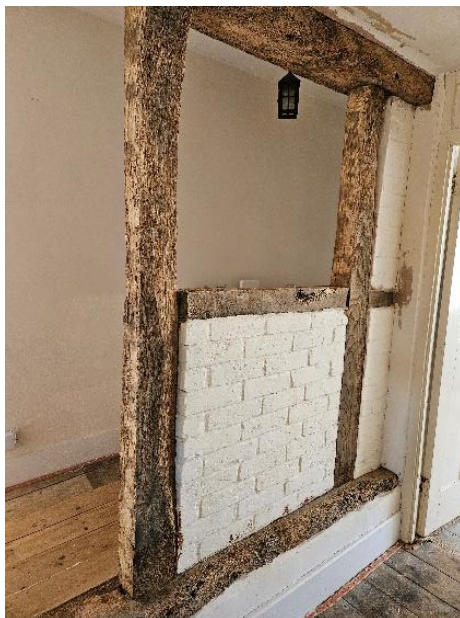
Fig.72 Stud wall in passage
