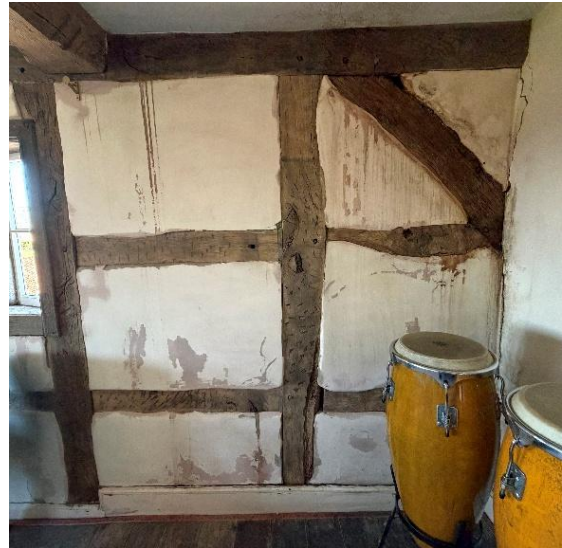
Fig.77 Front wall jowelled post, long straight brace, near-square panels
