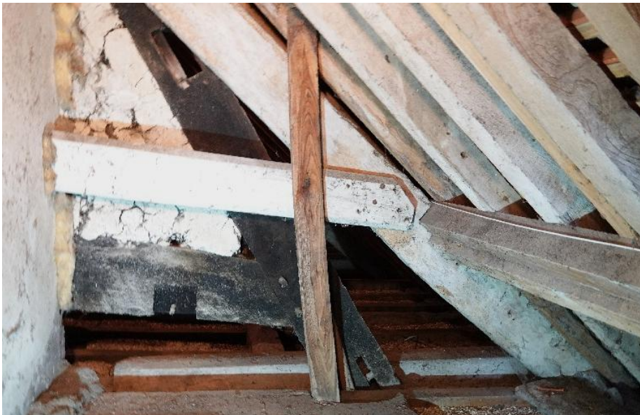
Fig.117 Truss T2 from the NE. This view shows T2A with its nailed-on collar
