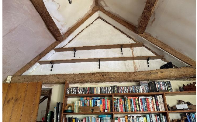
Fig.40 Study (G3) looking towards the hearth Fig.41 North-west end truss
