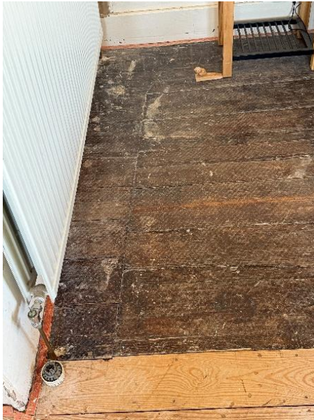
Fig.79 Former alignment of landing partition reflected in floorboards
