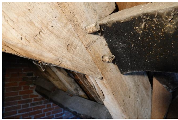
(left) Fig. 139 A re-used rafter pair in the crosswing roof. (Right) Fig. 140 Gouge marks on T5
