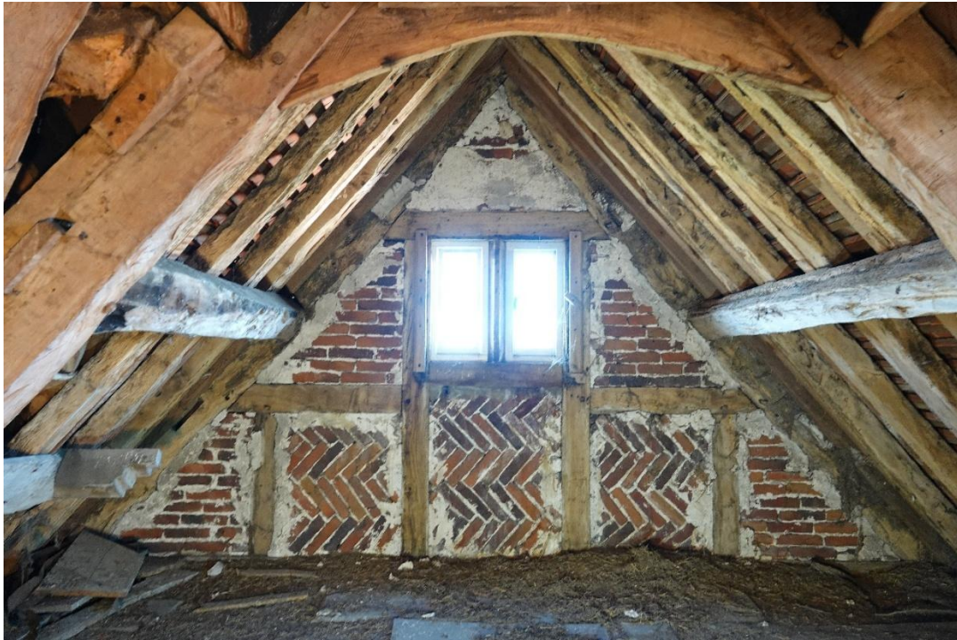
Fig.147 The timber-framing of the front (NW) gable, set in truss T6
