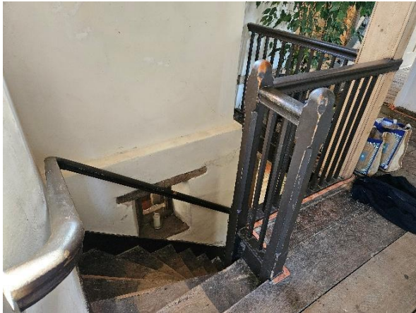
Fig.62 Looking south-east. Stair balustrade, with stop-chamfered newel posts
