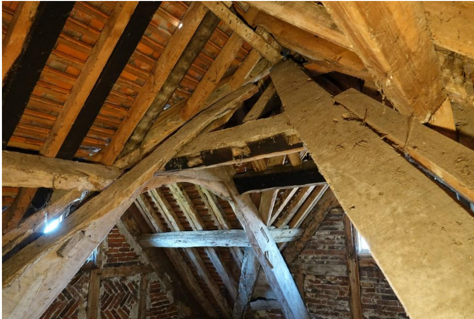
Fig. 149 The valley boards from the hall side (SW)
