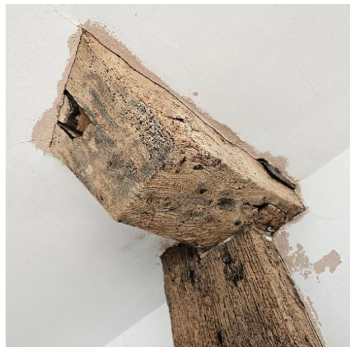
Fig.101 Post and stub-tie
