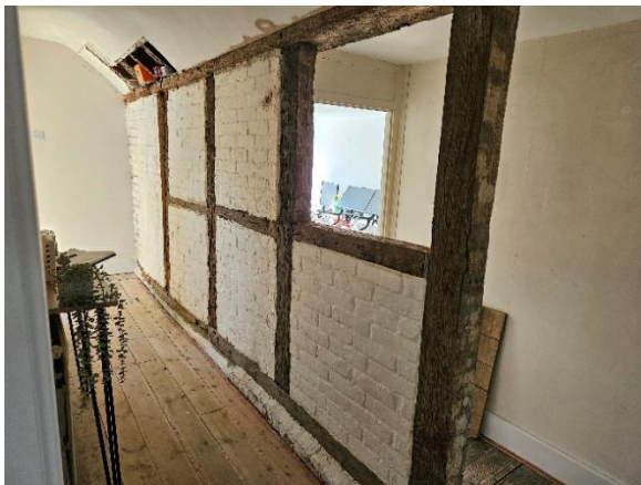
Fig.95 Rear corridor, looking south-west
