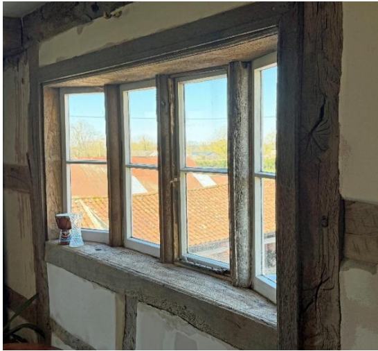
Fig.83 Timber 4-light oriel window, with ovolo-moulded mullions, ledge and soffit Fig.84 Original setting-out marks on stud; architrave added later, nailed
