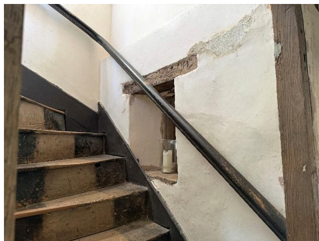
Fig.32 Inserted 18 th century window lighting stair
