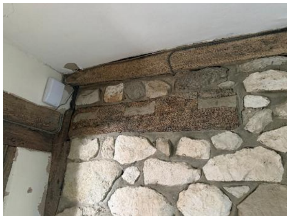
Fig.10 Embedded beam with joist pockets
