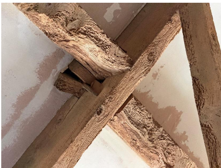
Fig.42 Staggered butt purlins with tusk tenons
