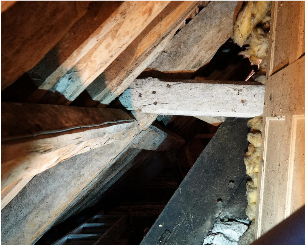
Fig.131 This view shows the nailed collar on T2A
