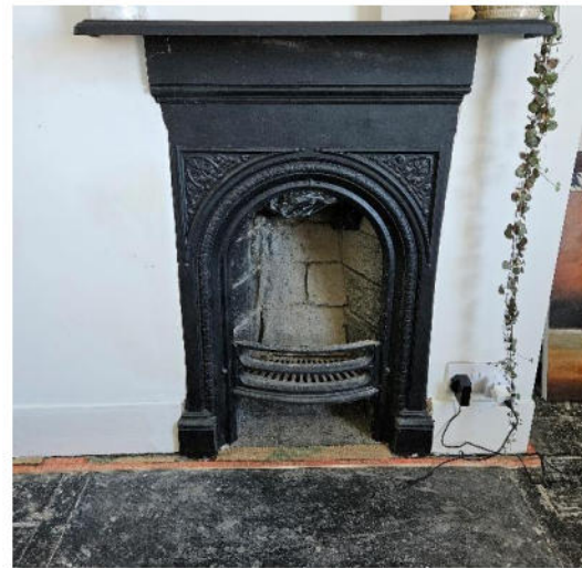
Fig.110 Arched register grate
