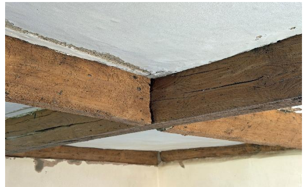
Fig.54 Nailed junction of beams
