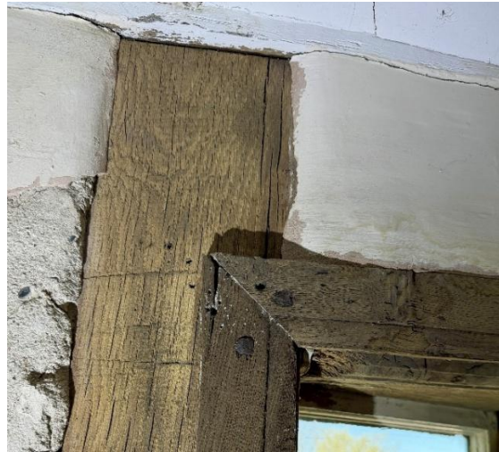
Fig.83 Timber 4-light oriel window, with ovolo-moulded mullions, ledge and soffit Fig.84 Original setting-out marks on stud; architrave added later, nailed
