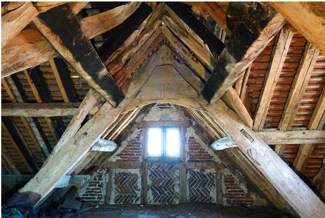
Fig.138 Truss T5 looking NW to the front wall
