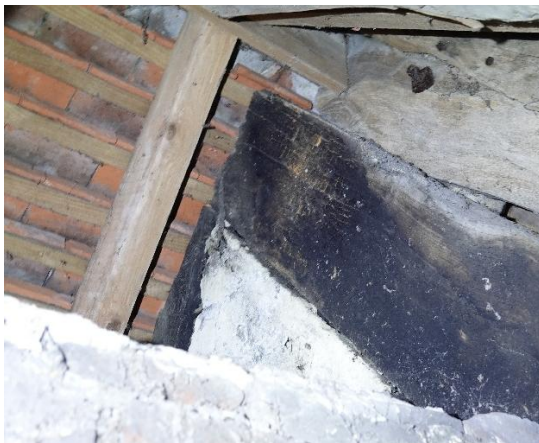
(left) Fig.119 Apex detail of T2 from the SW side; the far principal has been cut back by the later replacement tiled rafters. (right) Fig.120 Detail showing the staining of the principal and the sooting of the infill on the SW side
