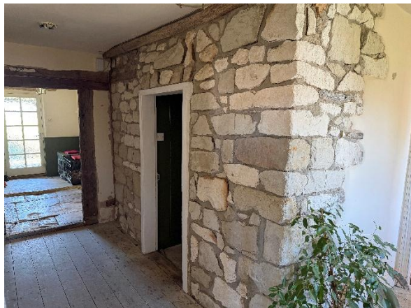
Fig.27 Modern partition to living room (G9). The visible beam butted against the former suggested smoke bay
