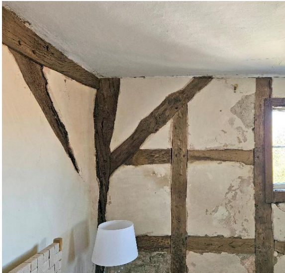
Fig.77 Front wall jowelled post, long straight brace, near-square panels
