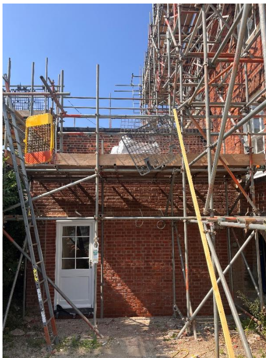
Photograph 3. Location of Installed Rooflights in Roof 7 (Table 1, Item 13)
