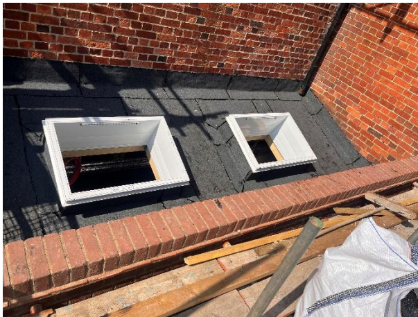
Photograph 2. Installed Rooflights in Roof 7 (Table 1, Item 13)
