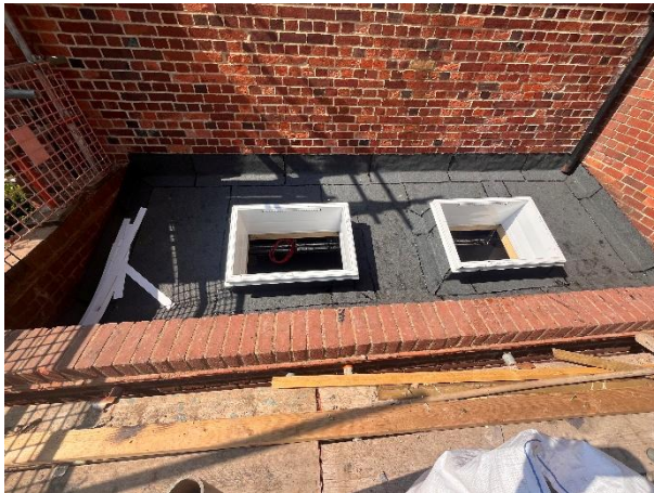
Photograph 1. Installed Rooflights in Roof 7 (Table 1, Item 13)
