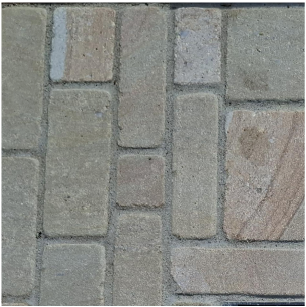
P3 Whixdale Sandstone Setts
