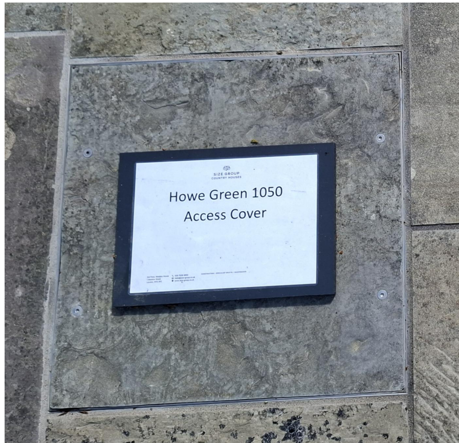
Recessed Manhole Cover
